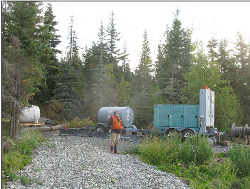
Figure III-1-3. Leveled genset pad from Spur Road extension.
