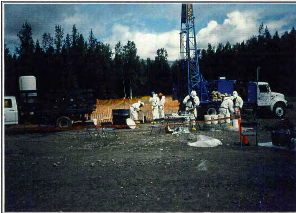
PHOTO 6: EOD specialist clears hole while geologist collects sample and split-spoon is cleaned.
