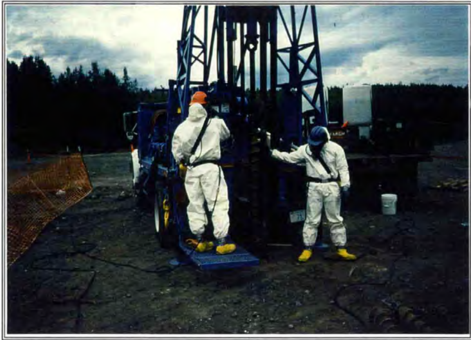
PHOTO 3: Drillers hammer split-spoon to collect first sample from boring.
