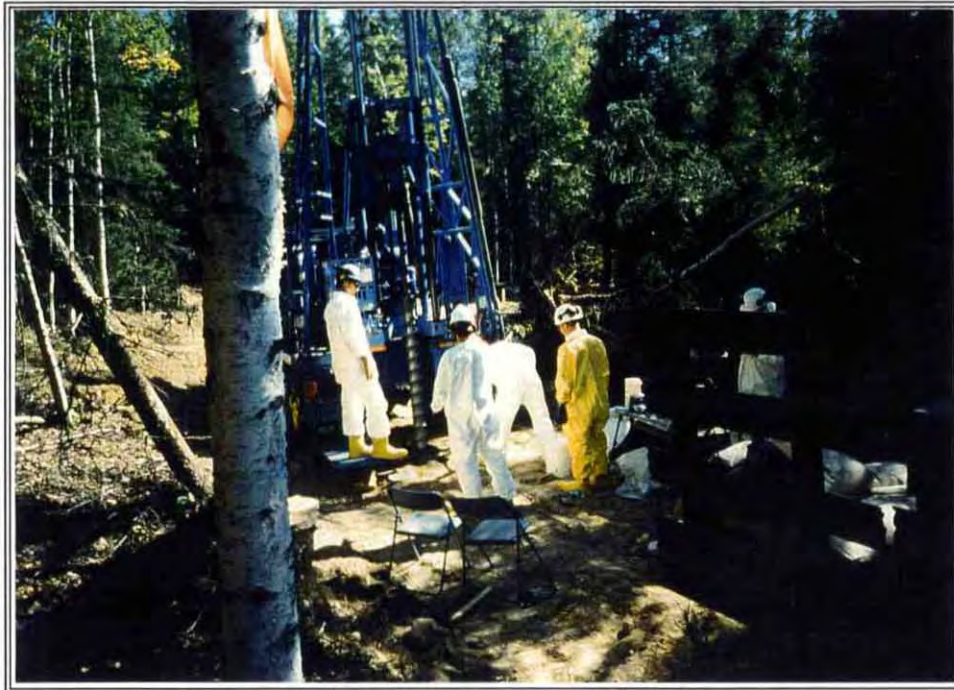
PHOTO 9: Drilling soil boring while in Level D PPE.
