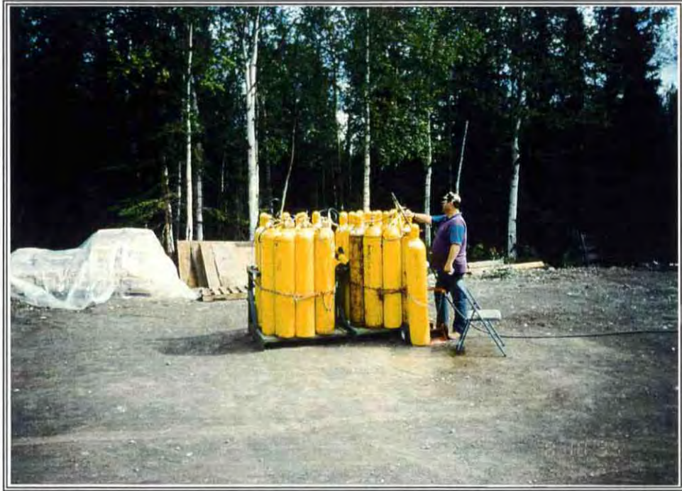
PHOTO 7: Health & Safety Officer checks pressure in supplied air tanks.
