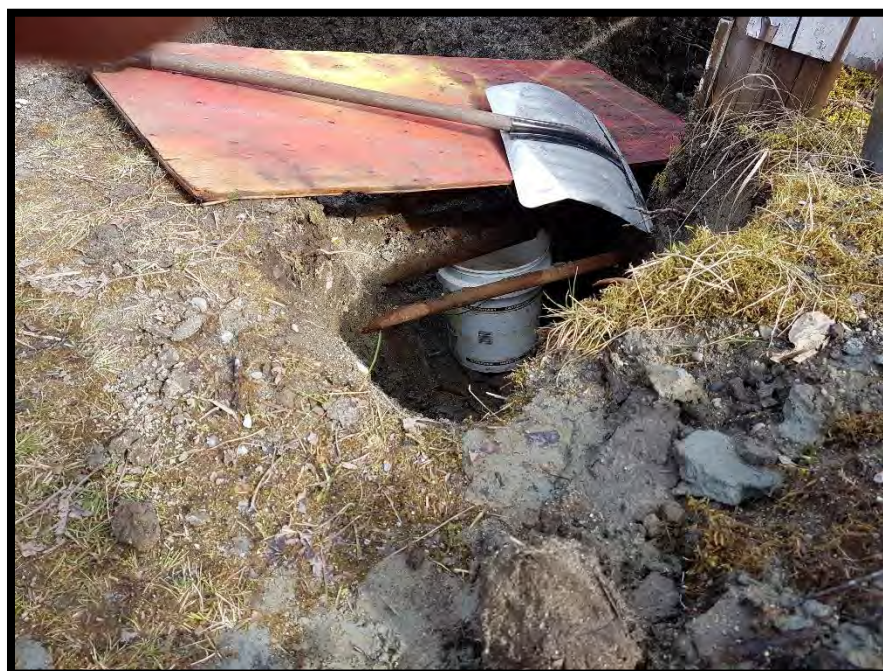
Photo 2: A five gallon bucket is placed under the leaking pipe(s) to capture fuel.
