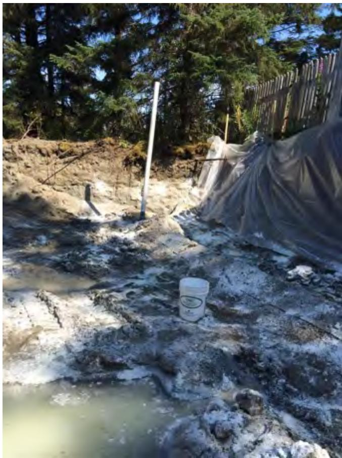
Photo 7: Extent of Excavation with groundwater interface drain, ORC and side curtain
