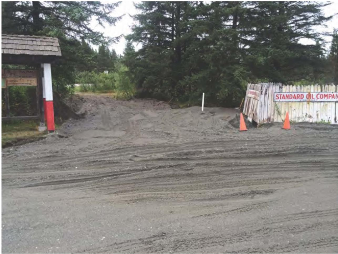
Photo 11: Filled excavation. Groundwater interface access at white standpipe
