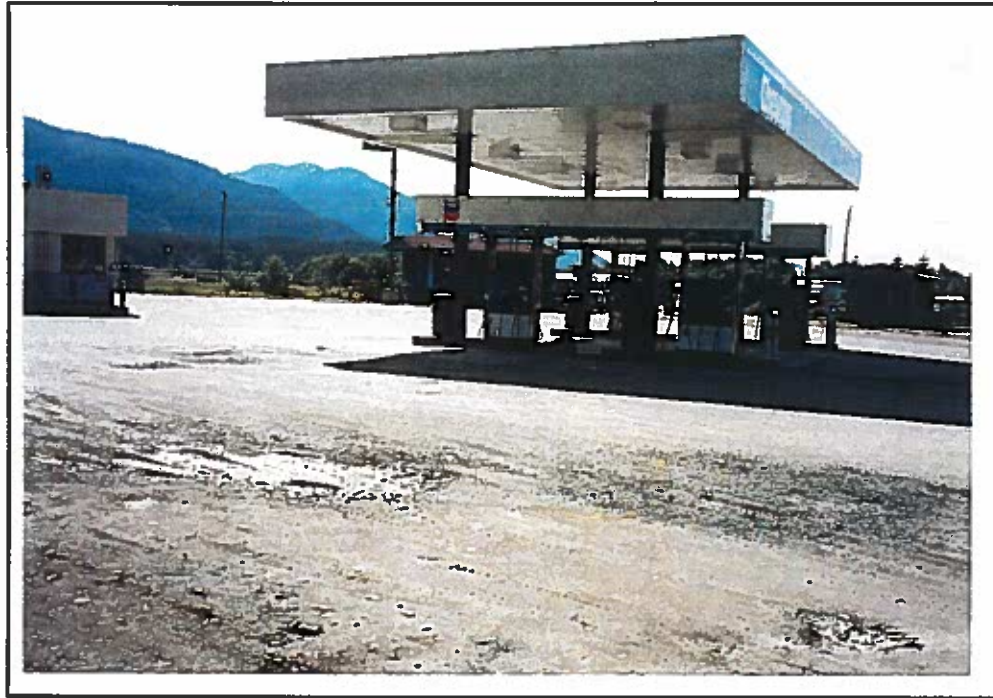
New pumps, with site of former tanks in foreground.
