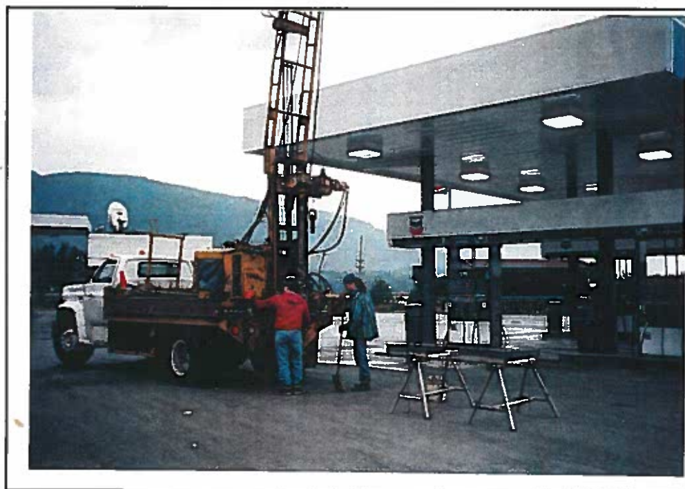
Setting up to drill Test Hole #1, 8/30/94
