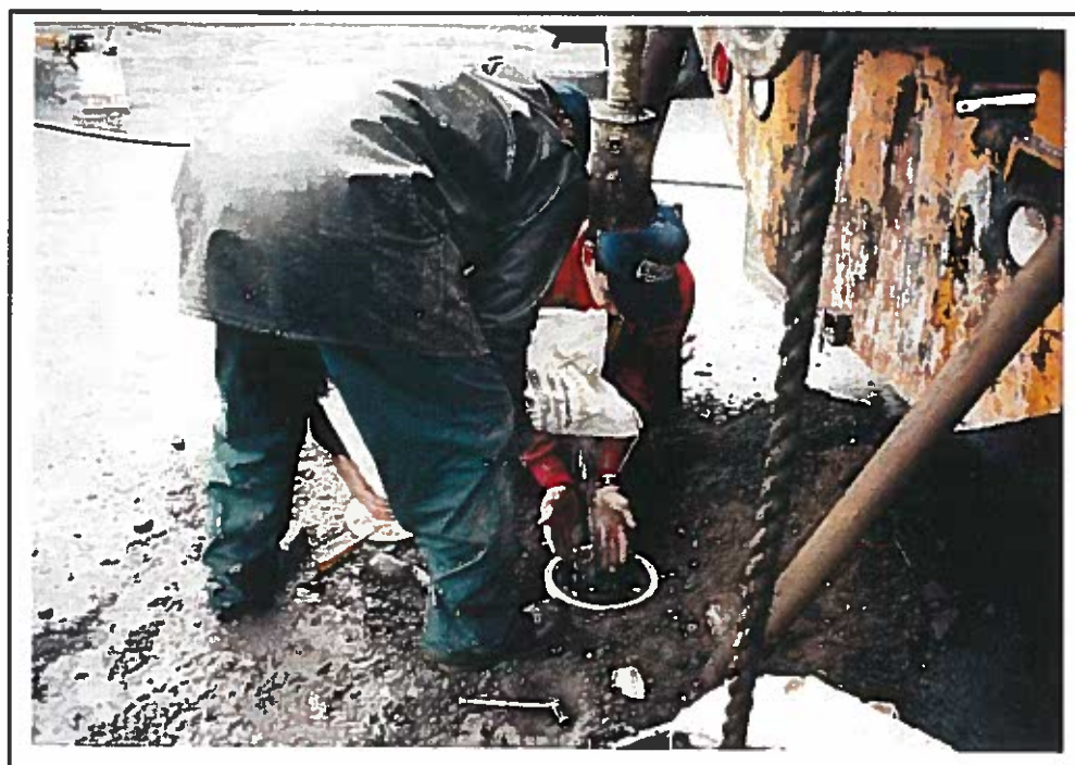
Installing water monitoring well.
