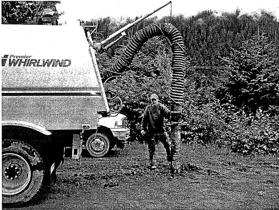
Whirlwind cleaner digging last of MW-2
