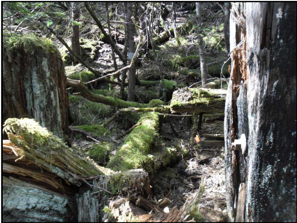
Photo 8: Looking north through the wooden timber foundation remnants at sample location NMM-08.
