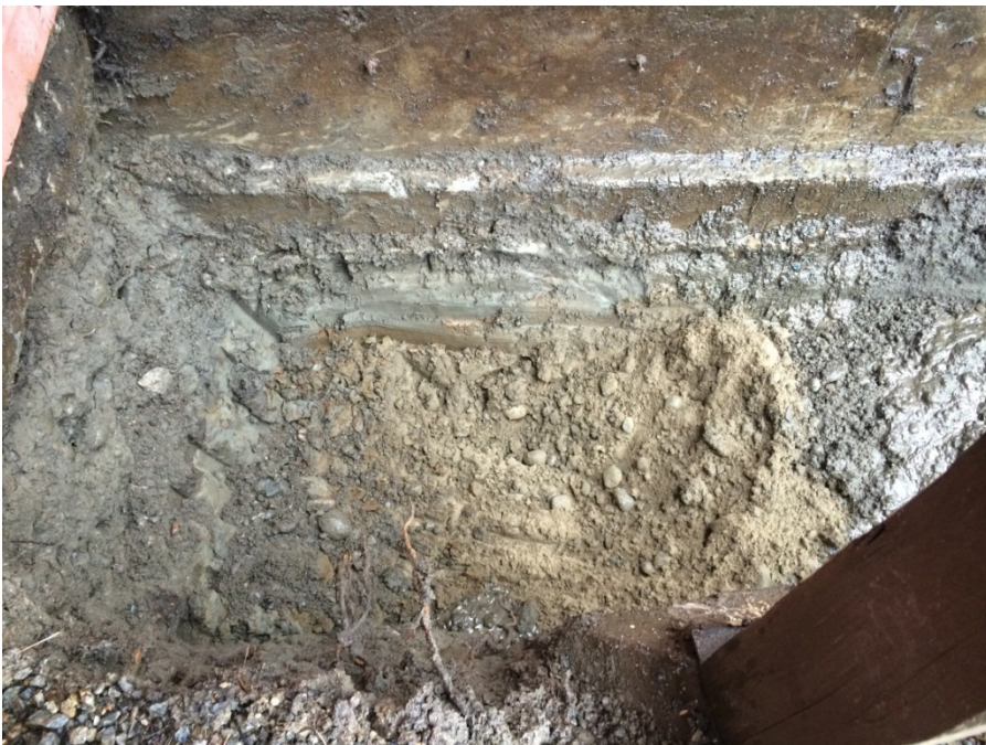
Photograph 4 - TP1: grey silty sand visible from approximately 3 feet to 6 feet followed by brown sand and gravel with cobble (>6 feet).
