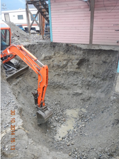
Photograph 7 - "Area 2" excavation looking northwest. Groundwater seepage at approximately 13.5 feet below grade.
