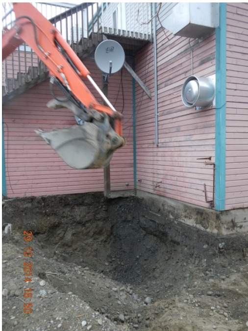
Photograph 6 - "Area 2" excavation looking north. Dark grey hydrocarbon-like staining visible at the location directly below the former ASTs.
