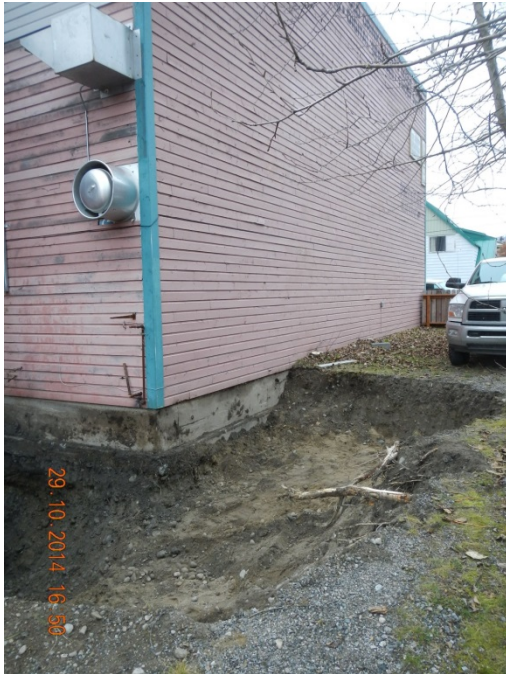
Photograph 5 - "Area 1" excavation on the neighboring property looking north.
