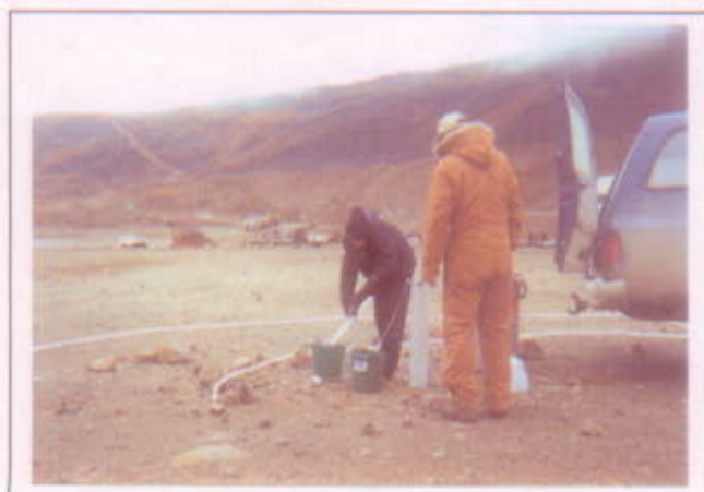
Purging groundwater prior to sample collection at well WW-02, SS15.
