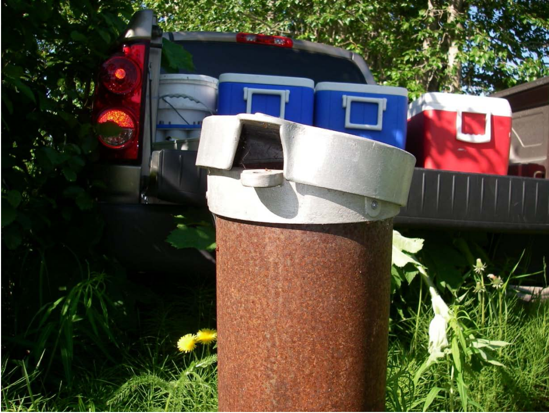
Photo 5: AP-3503, looking W; note cock-eyed lid due to inner casing jacking
