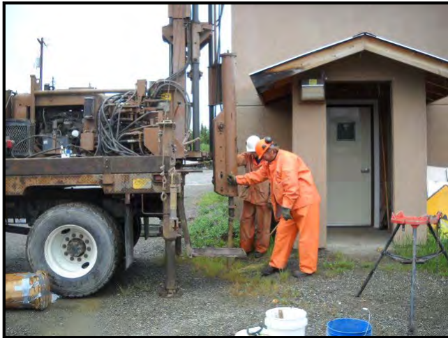
Boring B-2, looking Southeast.
