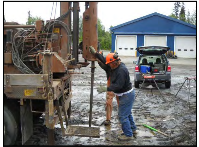
Boring B-2, looking East.
