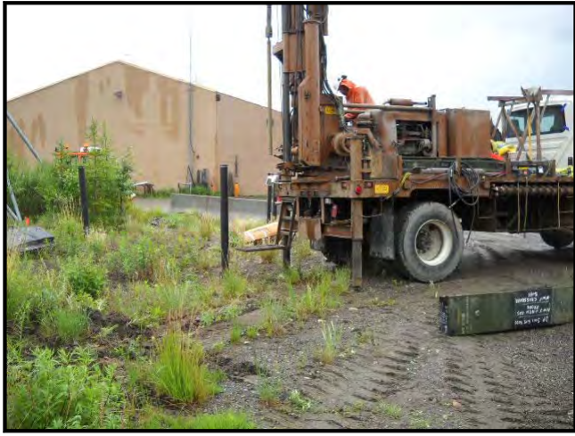
Boring B-1, looking South.
