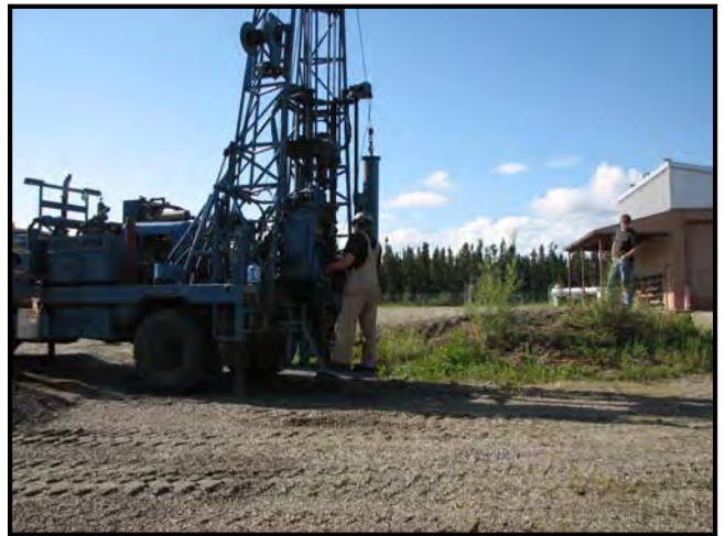
Boring B-2, looking South.
