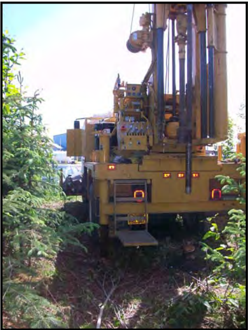
Boring B-1, looking South.
