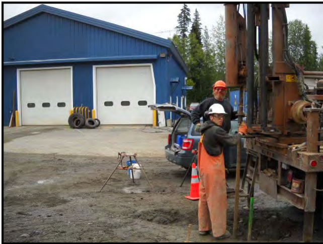
Boring B-1, looking East.
