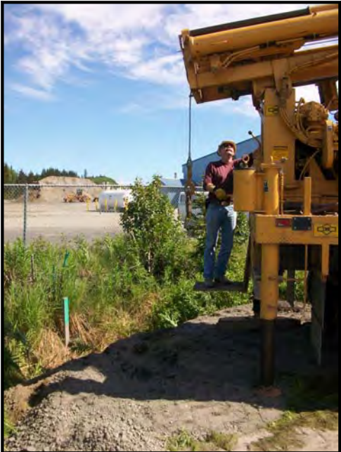
Boring B-2, looking Southeast.
