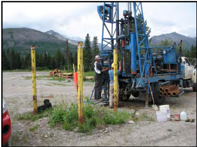
Boring B-1, looking Southeast
