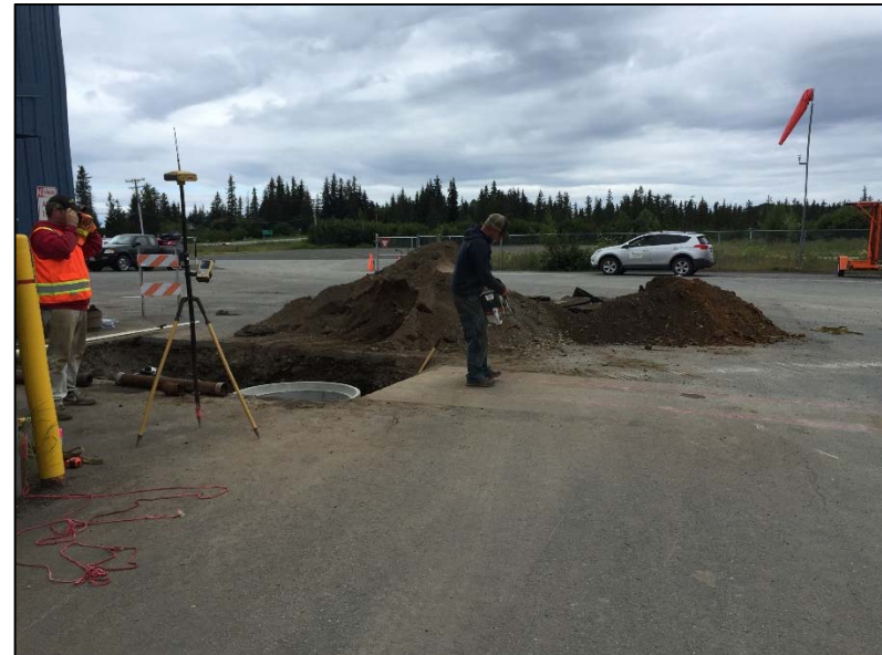
Lift Station Stockpiles: Stockpile A (left) and Stockpile B (right) (7-11-16)
