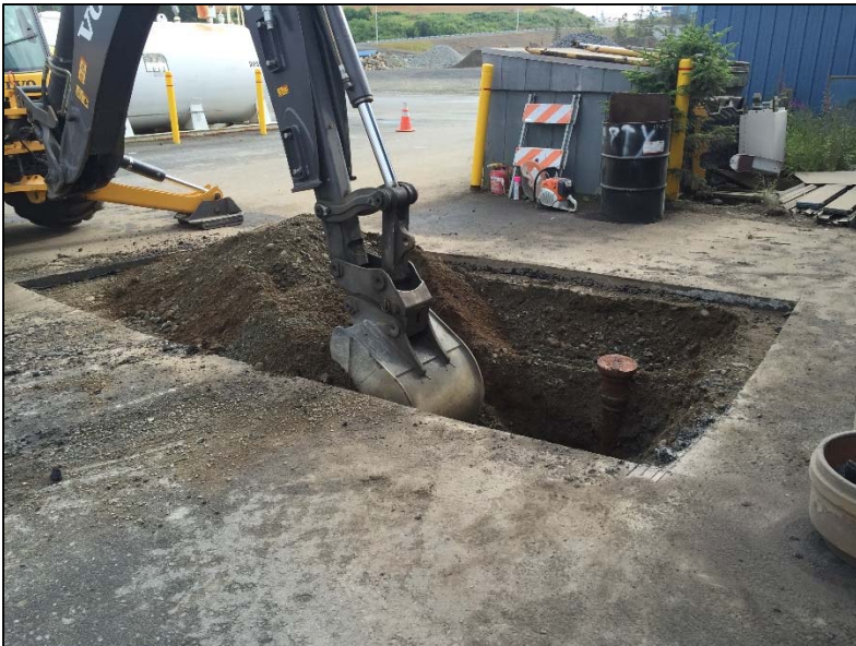
Lift Station Excavation, view northeast (7-11-16)
