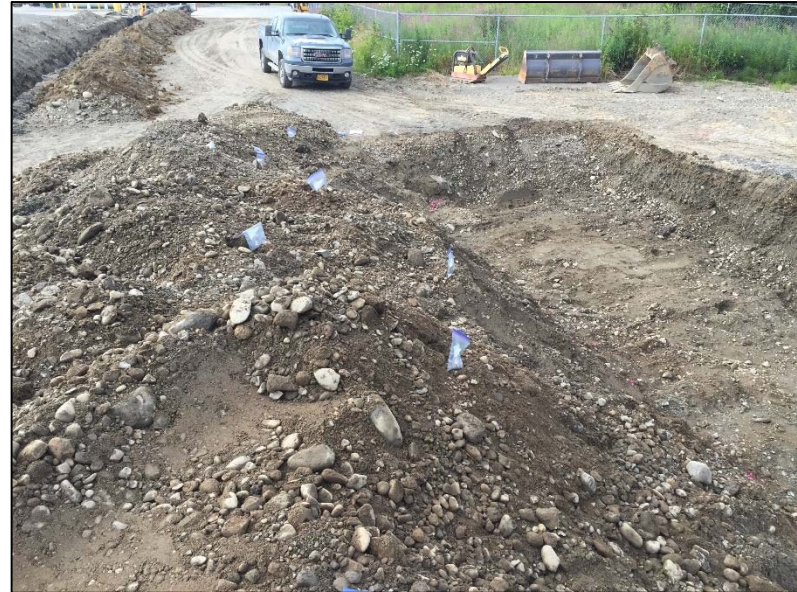
Retention Pond Excavation, view south (7-12-16)
