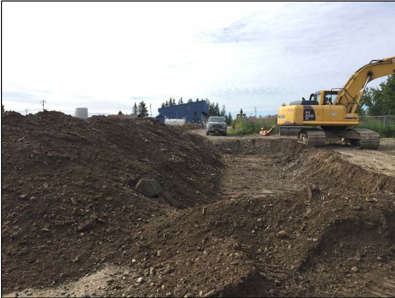
Retention Pond Excavation, view south (7-12-16)
