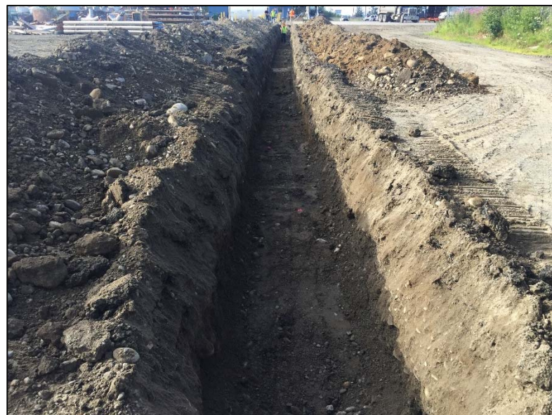
Water Line Trench excavation, view south (7-11-16)
