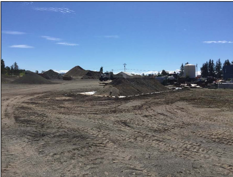
Segregated stockpiled soil, view southeast (7-12-16)
