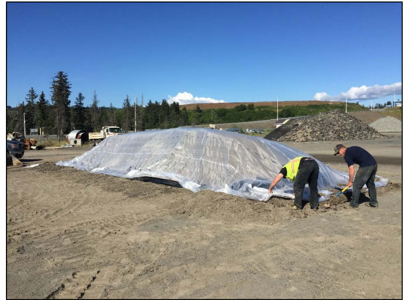
Segregated stockpiled soil covered, view northeast (7-12-16)
