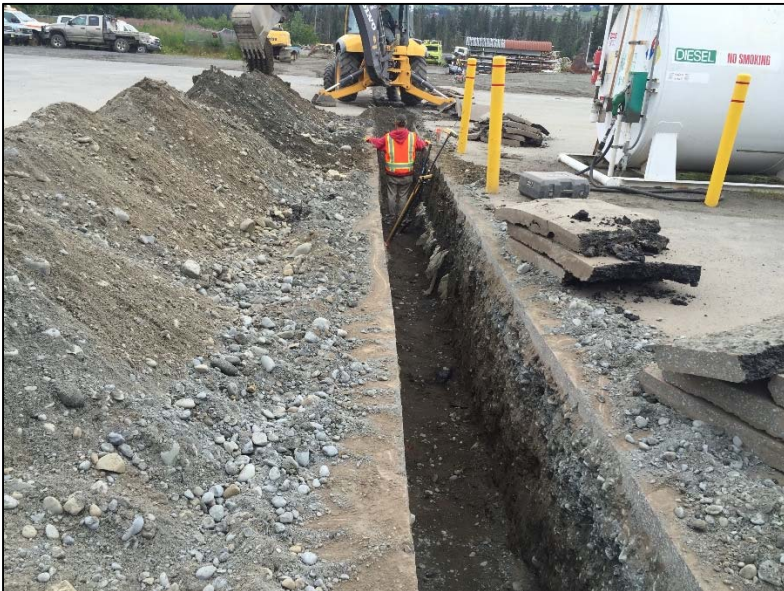
Water Line Trench excavation, view north (7-11-16)
