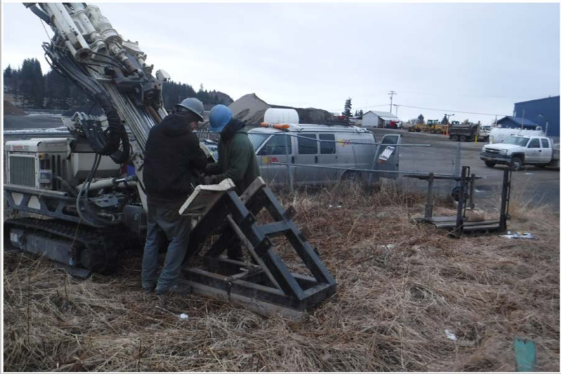
Photo 3: Drilling at work site. 2/18/2016
