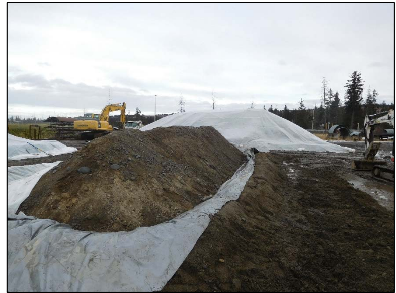
Stockpile with the visqueen cover removed
