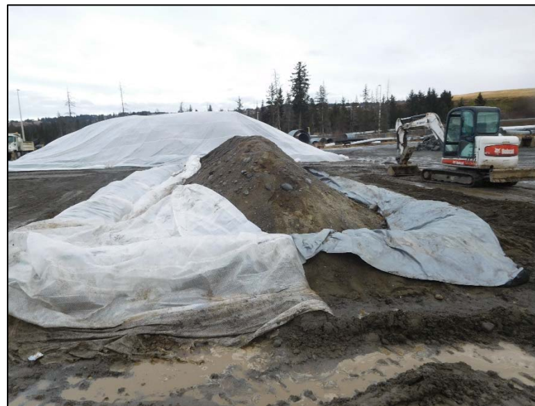
Visqueen being replaced over stock pile once sampling is complete
