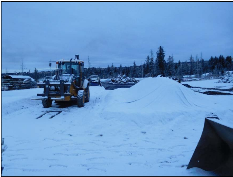
Stockpile covered with visqueen in secondary containment
