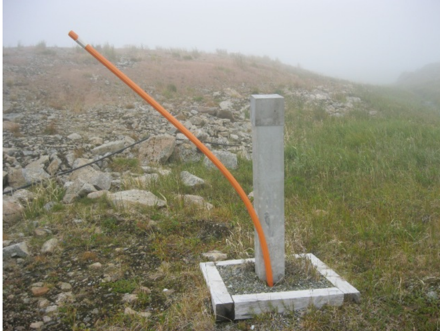
Photo No. 29 – 20 August 2012 LF003 Landfill No. 2; CMW2; view looking south.
