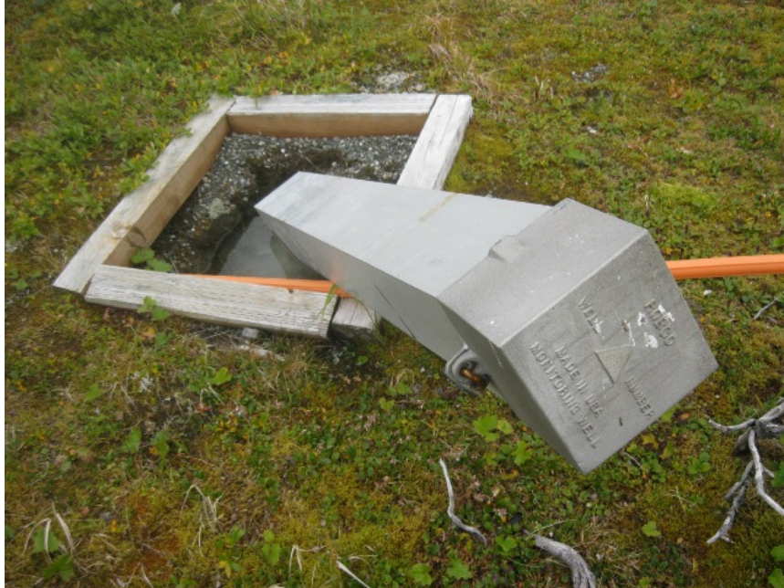
Photo No. 24 – 20 August 2012 LF003 Landfill No. 2; CMW7; view facing northeast.
