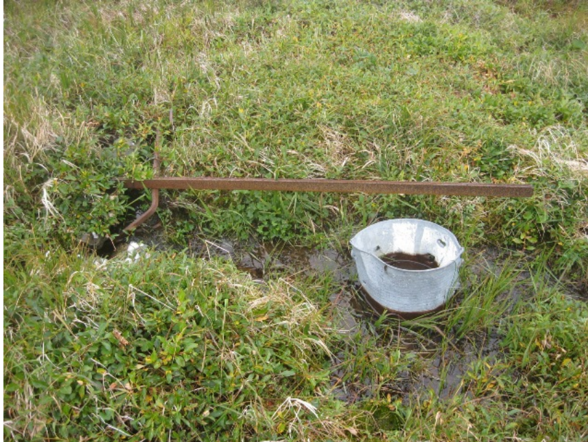
Photo No. 25 – 20 August 2012 LF003 Landfill No. 2; debris located at south end of site.
