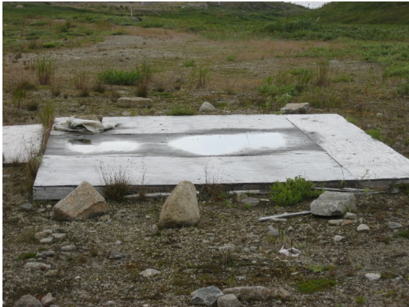
Photo No. 14 – 20 August 2012
