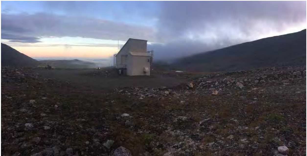
SS017 view west. Lower tram building shown.
