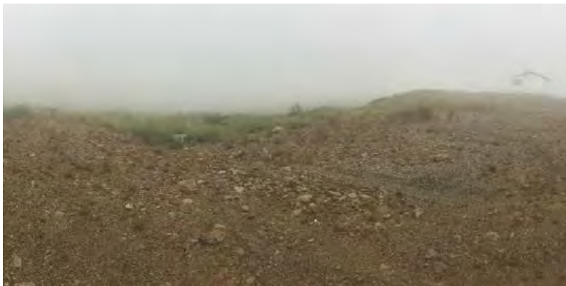
SS010 view west. MW3 shown at photographs left. Former tank pad shown on the right.
