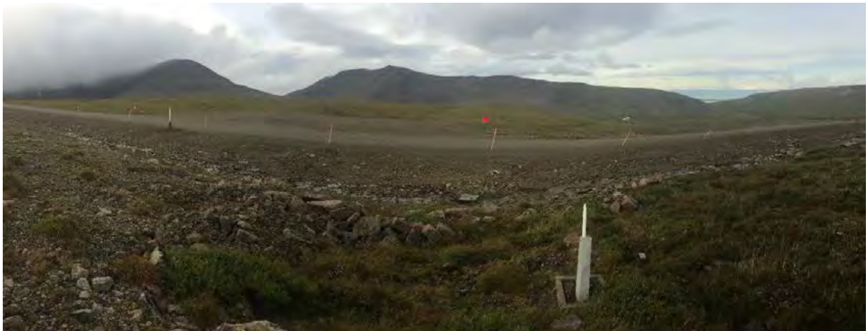
LF003 view south. CMW3 in foreground with MW-2 and LUC signage in background over landfill cap.
