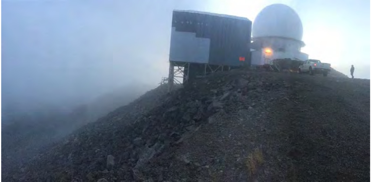
SS016 view north. LUC signage (orange) shown mounted to the upper tram building.
