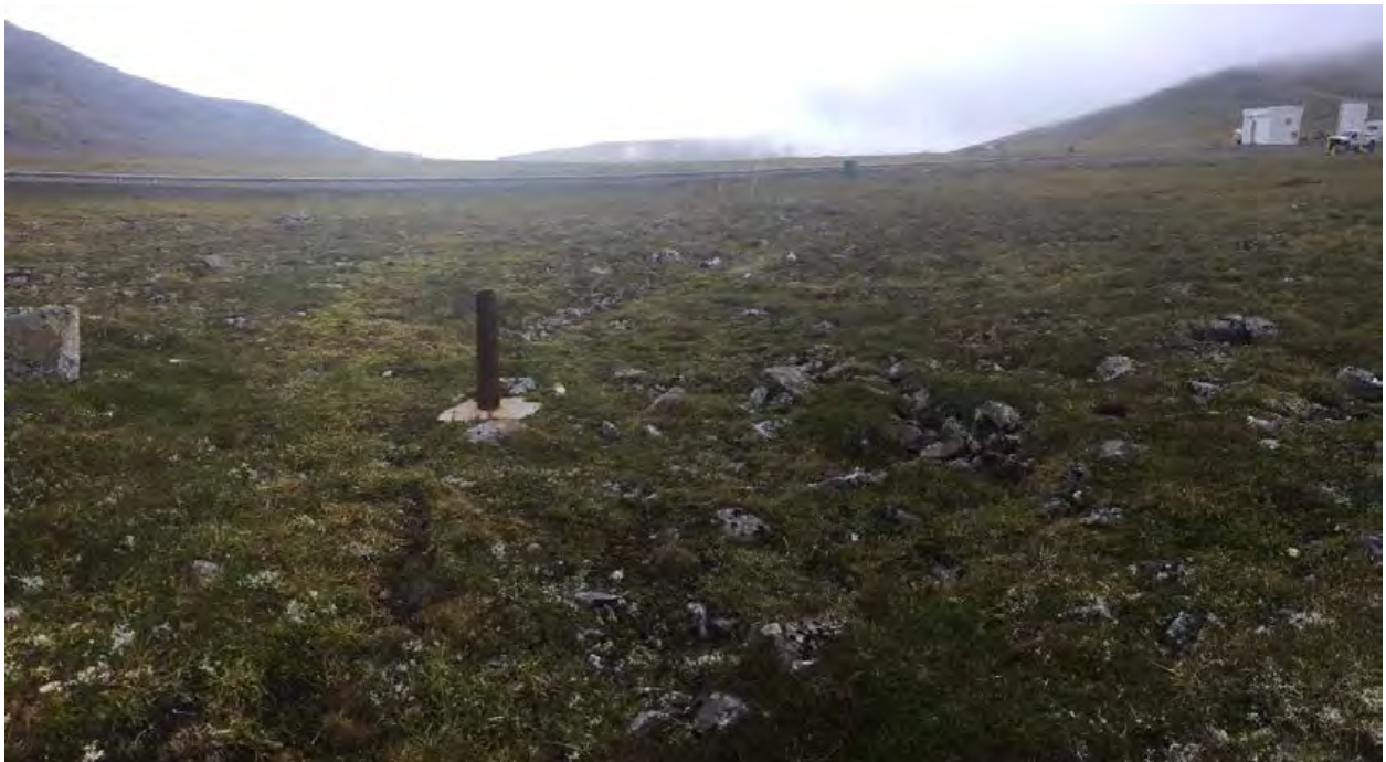
Site SS015 view south west. WW6 shown in foreground. Water transmission line pad and pump building shown in background.
