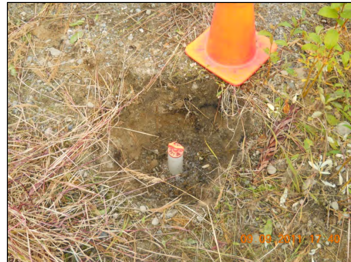
Typical Monitoring Well Installation – Missing Protective Casing
