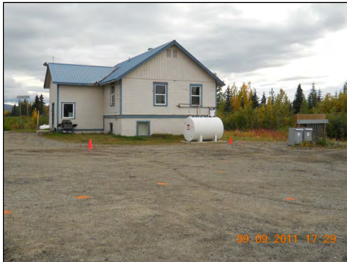
Hurricane Section House
