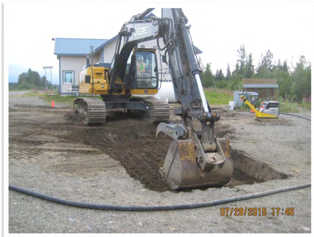
Photograph 10 – Active backfilling of the first North Excavation. View to south-southwest.
