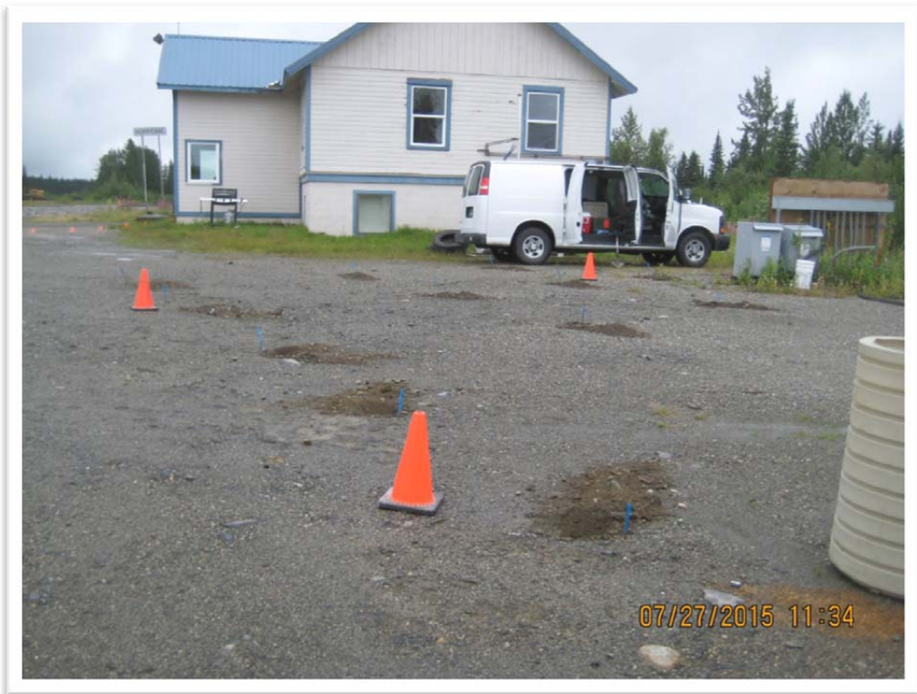
Photograph 2 – View of surface soil screening locations installed prior to excavation. View to southwest.
