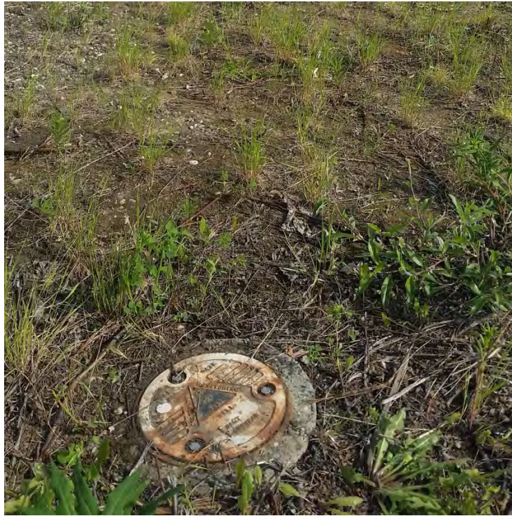
Photo 9: Unknown monitoring well “MW-A” located to the north of the FTP pond (June 5, 2018).
