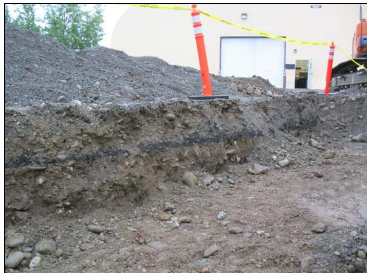
Asphalt layer contributing to DRO contamination found along the north end of the excavation at Building 17720.
