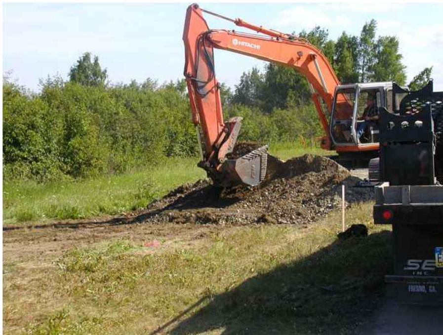
Photo 12. Temporary road removal.
