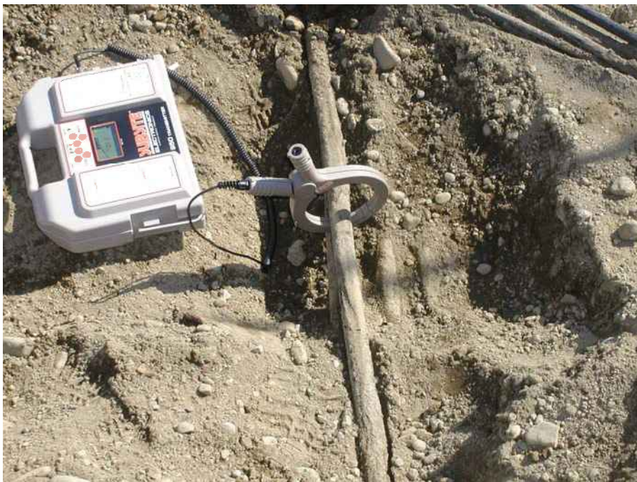
Photo 6. Testing cables for power.
