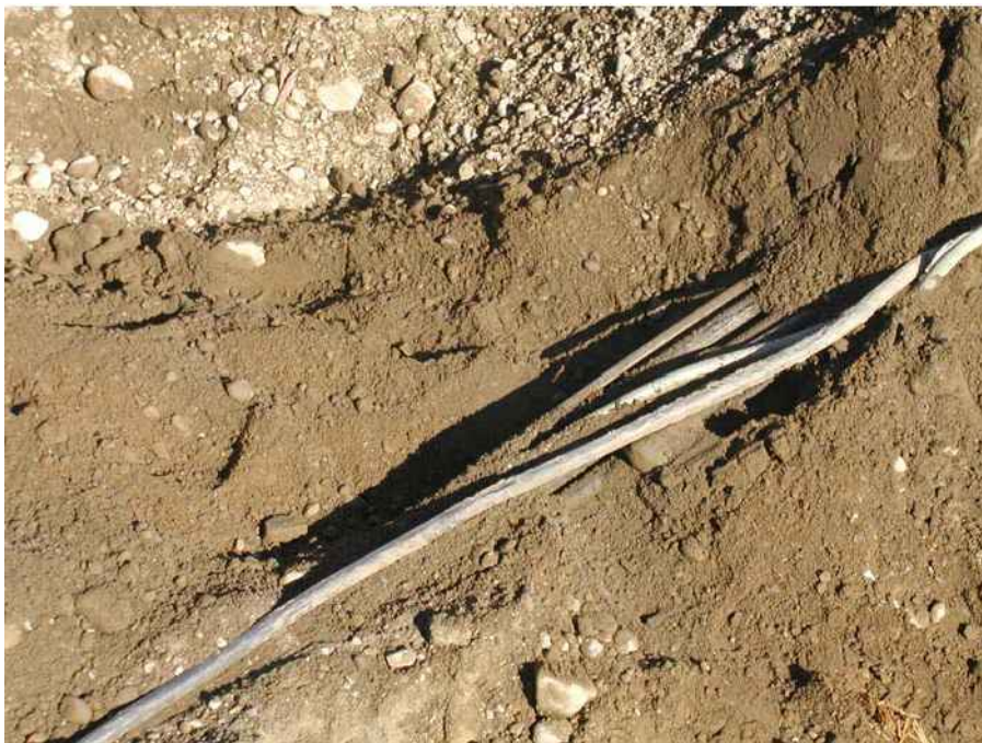
Photo 4. Cables exposed during excavation.
