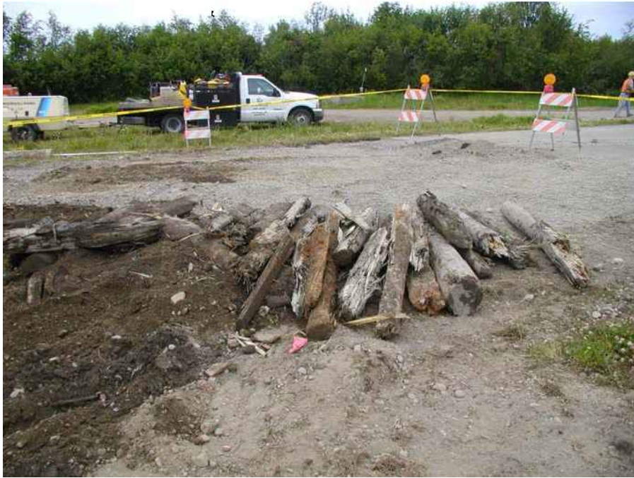
Photo 7. Debris removed from excavation.
