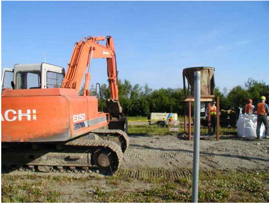
Photo 1. Initial site preparation - 20 June 2005.
