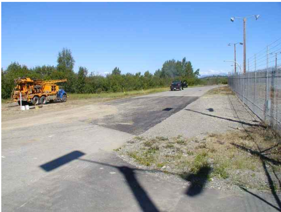
Photo 14. Paving complete and fence installed - 21 July 2005.
