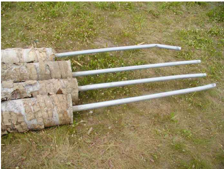
Photo 2. Fence and posts removed.
