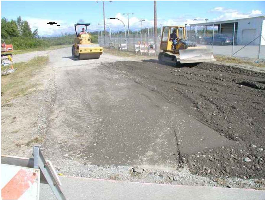
Photo 11. Compactor and dozer leveling the roadway.
