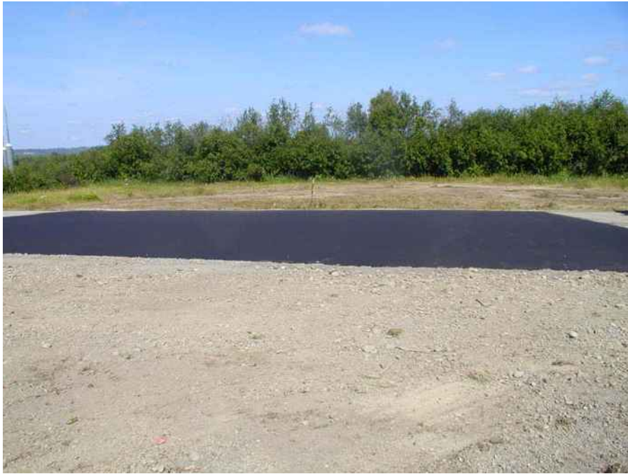
Photo 13. Roadway paving completed.
