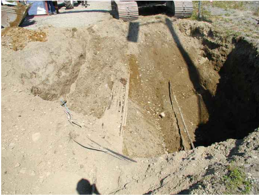
Photo 3. Cables exposed during excavation.
