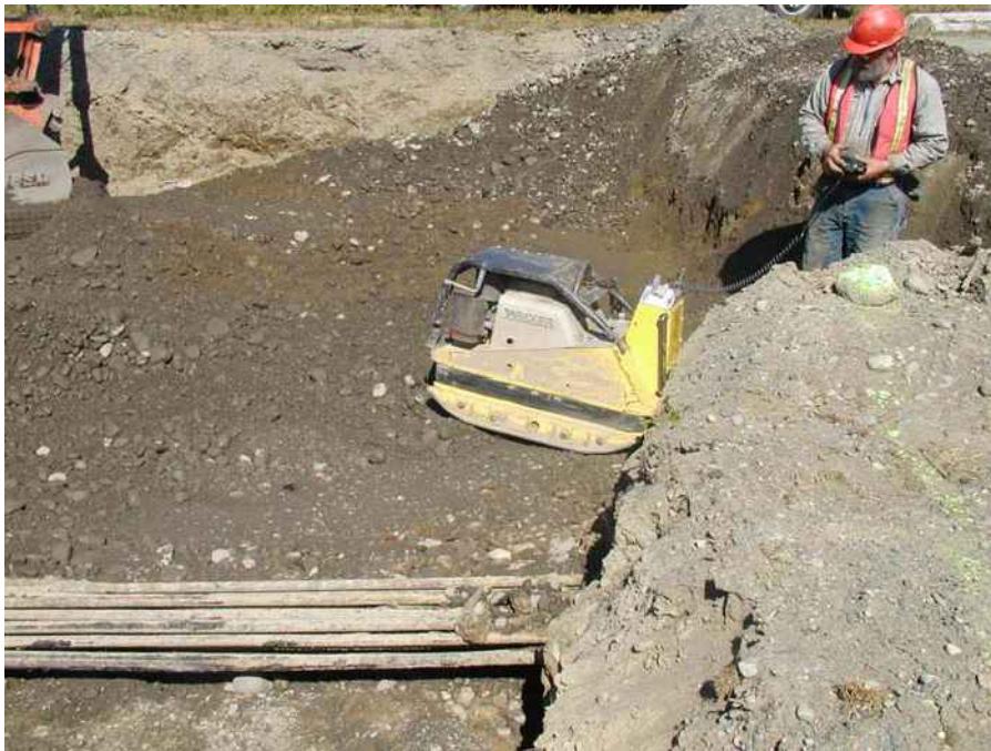
Photo 10. Vibrator compacting excavation backfill.
