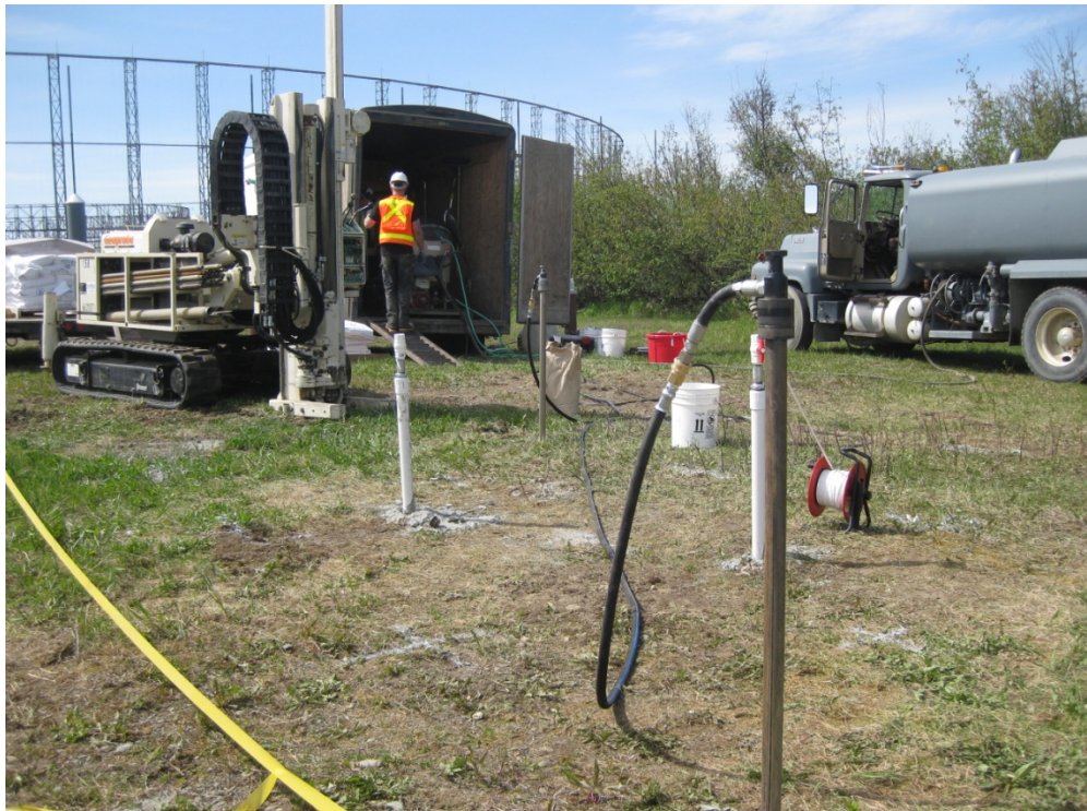
Figure 2.4 Injection into DPT Points at Test Cell No. 1
