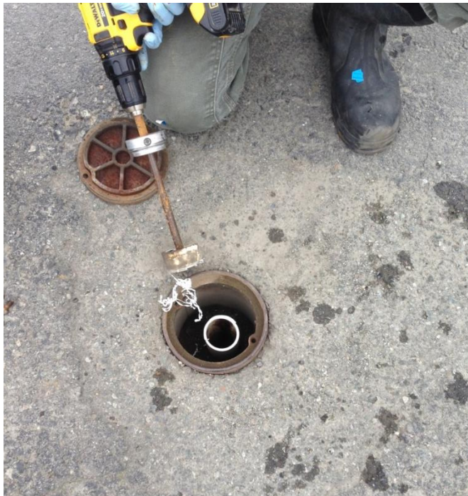
Photo 3: Maintenance at MW-6 included removing (cutting off) 1 inch from top of the well casing, so it was not hitting the monument cover.
