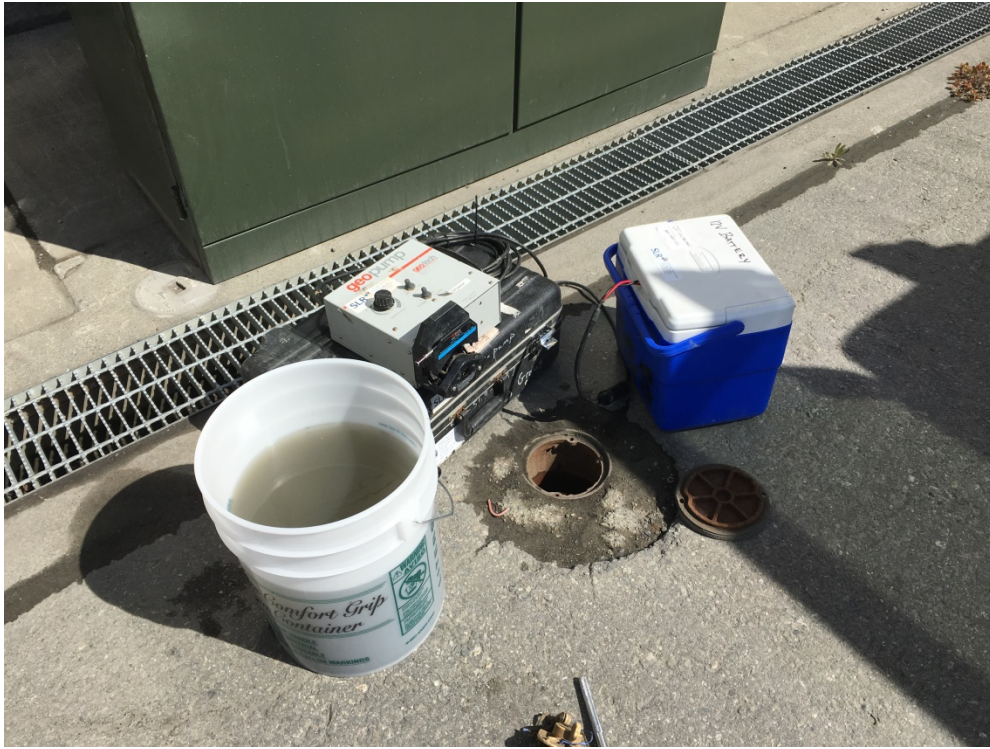
Photo 5: Monitoring Well MW-9 after purging on 6/13/16. Well was allowed to recharge and sampled on 6/15/16. Well located south of Transformer Shop
