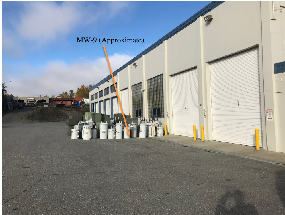
Photo 1: Transformer Shop building from the southeast. Approximate location of monitoring well MW-9 is shown.
