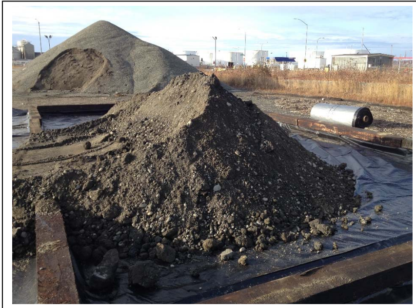
Photo 3: Looking west at approximately 25-cubic yard stockpile of contaminated soil placed on 20-mil petroleum resistant liner and surrounded by timbers. (October 24, 2014)
