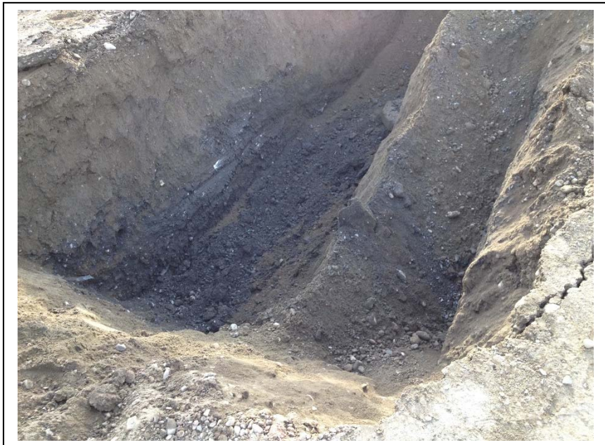
Photo 2: Looking southeast at the final depth of the TP-3/B-3 excavation. Note discolored soil in the lower portion of east sidewall. (October 24, 2014)
