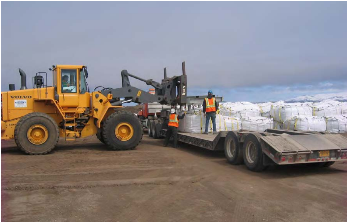
Photo 13: Unloading super sacks at the barge staging area, 2012
