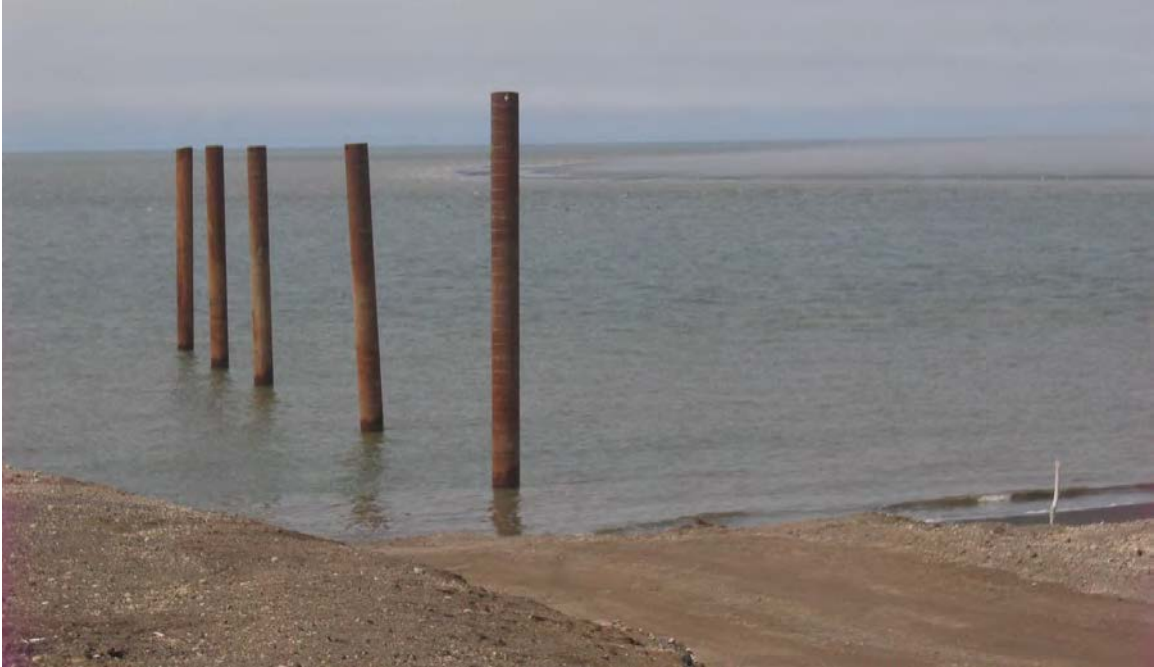
Photo 19: Steel pipe piling installed to provide mooring for barge, 2012
