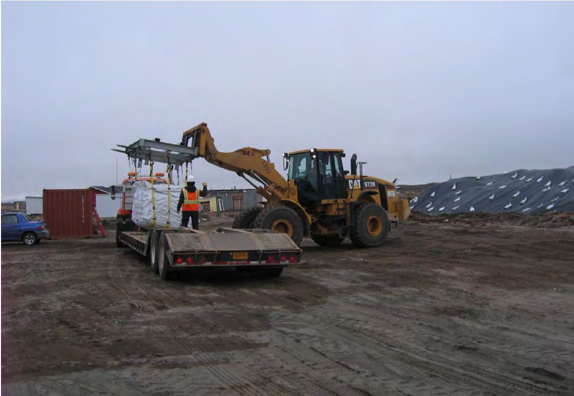
Photo 11: Loading low boy with 10-CY super sacks for transport to barge, 2012.
