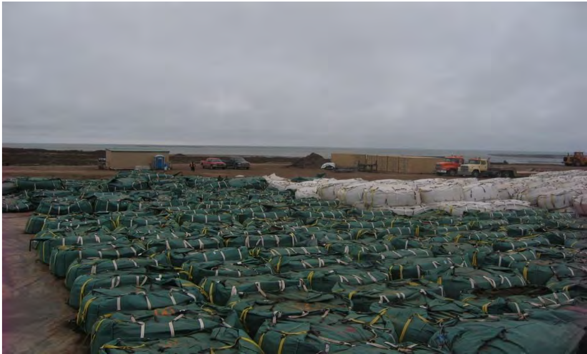
Photo 15: 5-CY and 10-CY super sacks of soil staged for barge loading, 2012.
