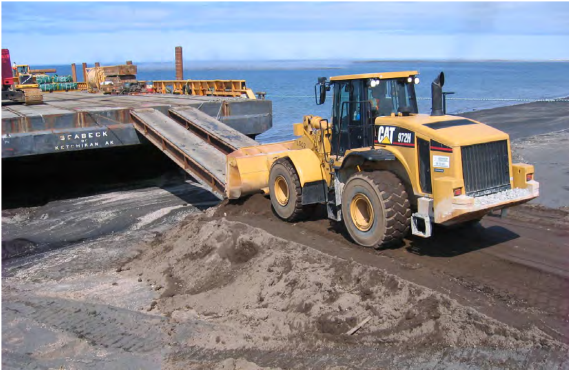
Photo 17: Constructing earth fill ramp to access barge, 2012
