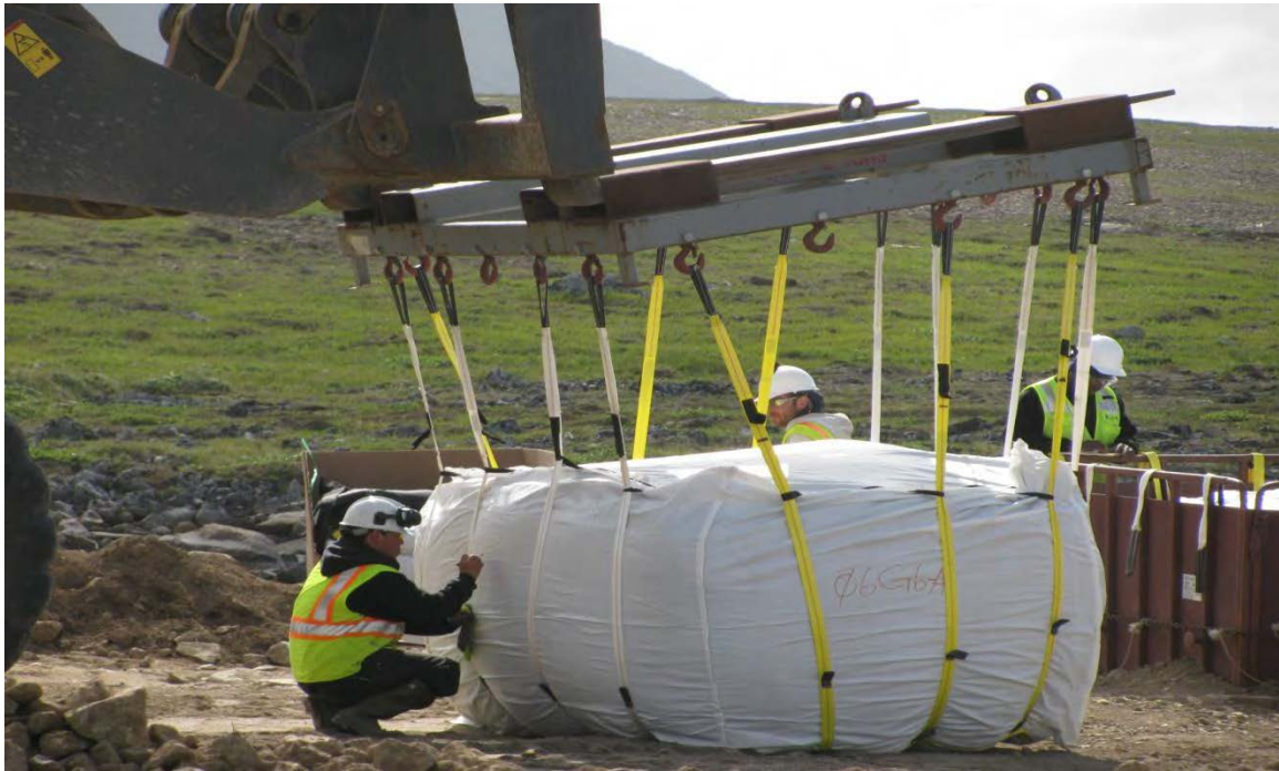
Photo 7: Labeling 10-CY super sack for waste tracking, 2013
