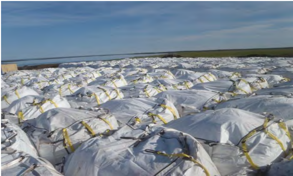
Photo 14: 10-CY Super sacks of unregulated waste soil staged for barge loading, 2012.
