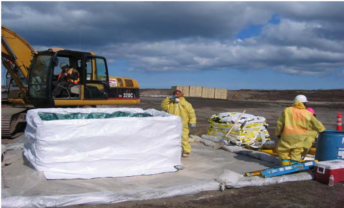
Photo 4: Super sack in loading frame prepared for filling with waste soil, 2012.
