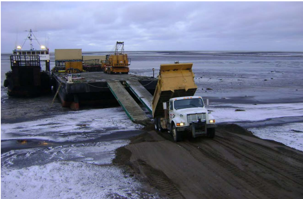
Photo 16: Constructing earth fill ramp to access barge, 2011
