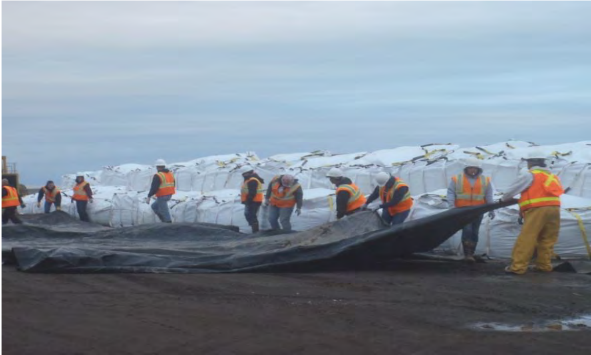
Photo 29: Covering super sacks for winter storage, 2012.
