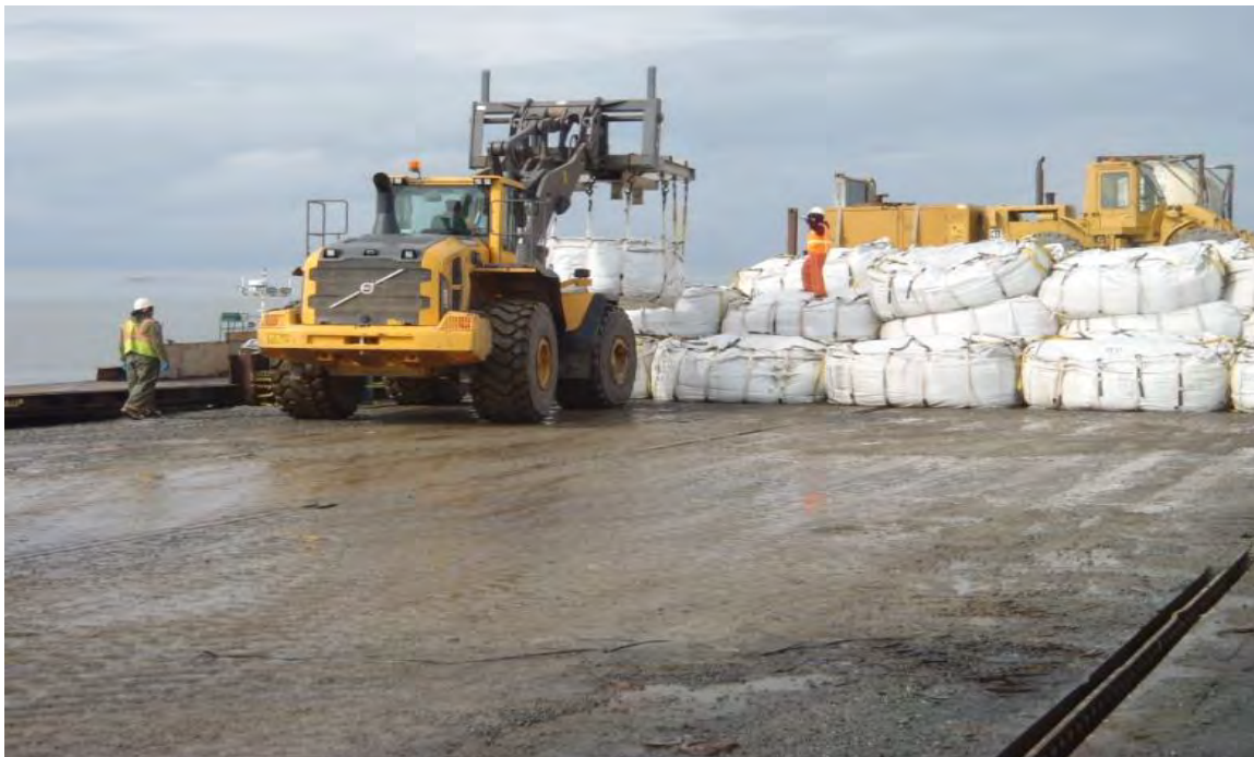
Photo 22: Stacking of 10-CY bags for transport on barge, July 2013.
