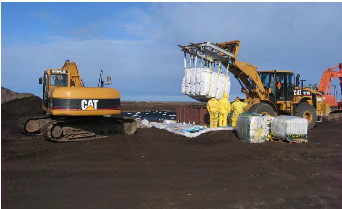
Photo 6: Lifting filled super sack from the loading frame, 2012.
