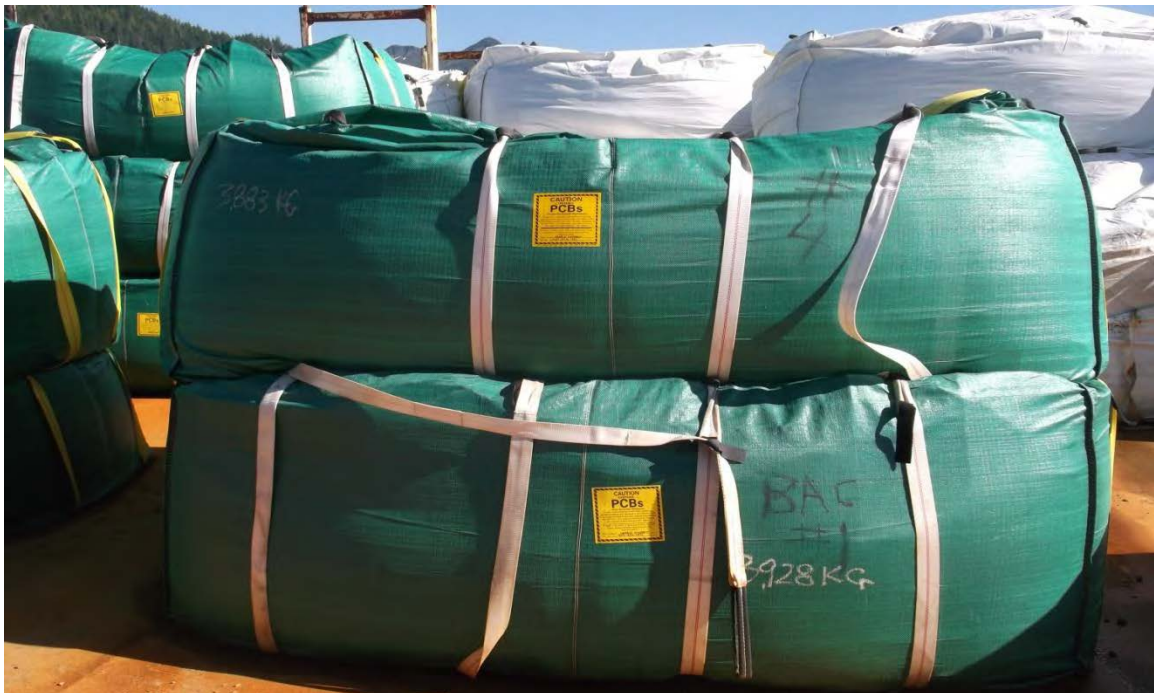
Photo 8: 5-CY Super sacks with PCB/Hazardous waste labels, 2012
