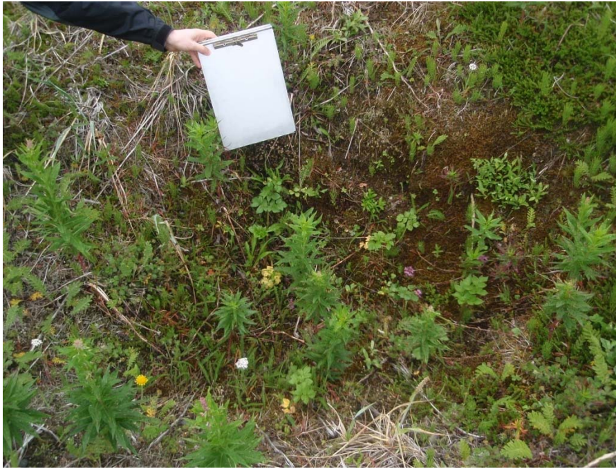
Photograph 9: LF007. Central portion of LF007 facing downward toward area of subsidence.
