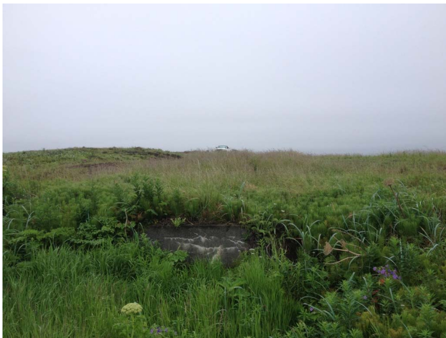
Photograph 6: SS004 outfall wing wall, facing southeast.
