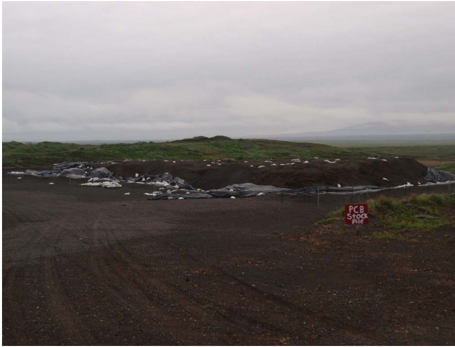
Photograph 3: OT001 - Uncovered PCB stockpile at the northeast end of OT001, facing northeast.
