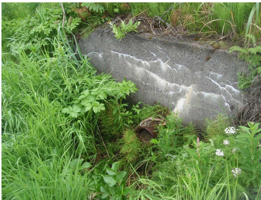
Photograph 7: SS004 outfall wing wall, facing east.
