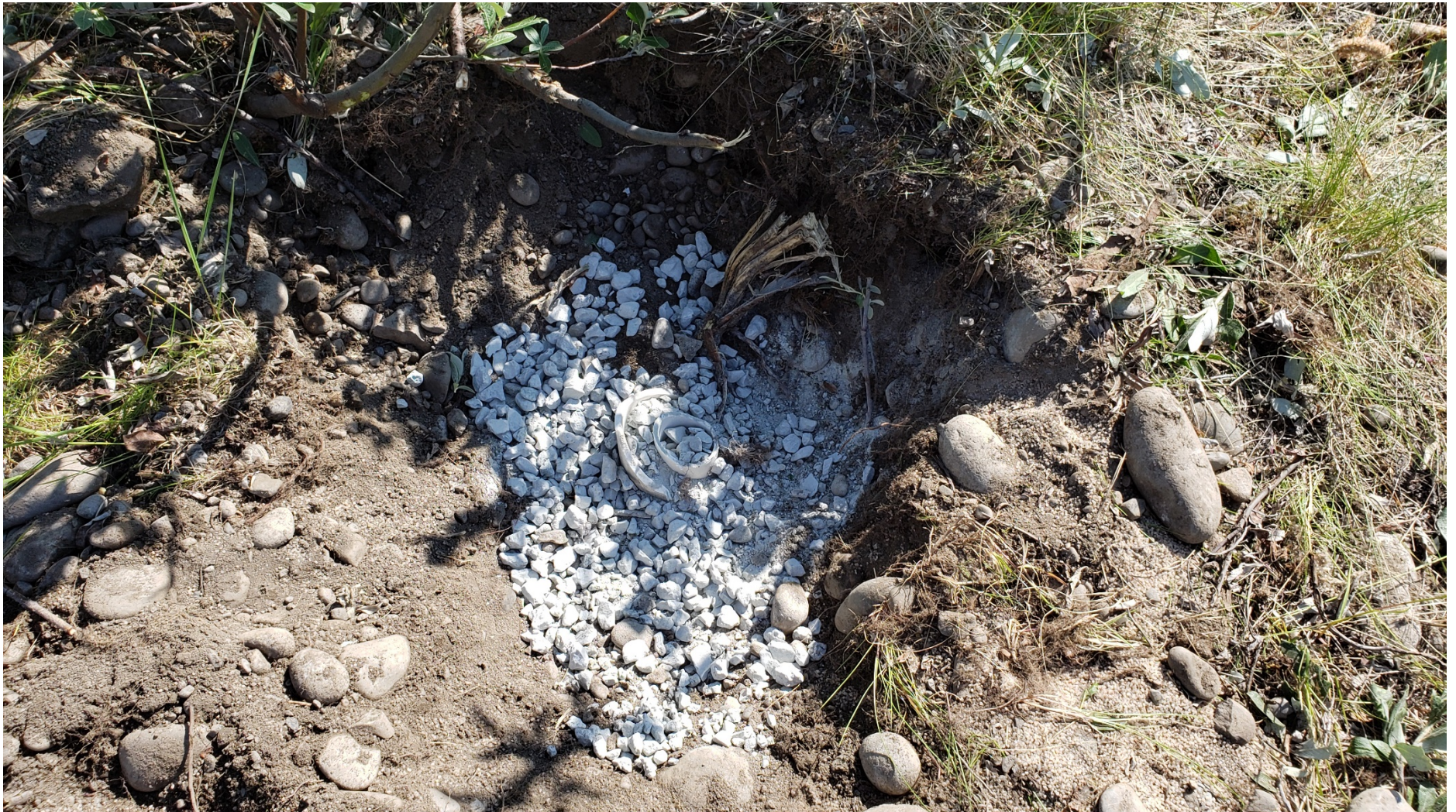
Photograph 2: Monitoring well Sentry-1R following removal of above-grade PVC and backfilling with bentonite chips (July 11, 2019)
