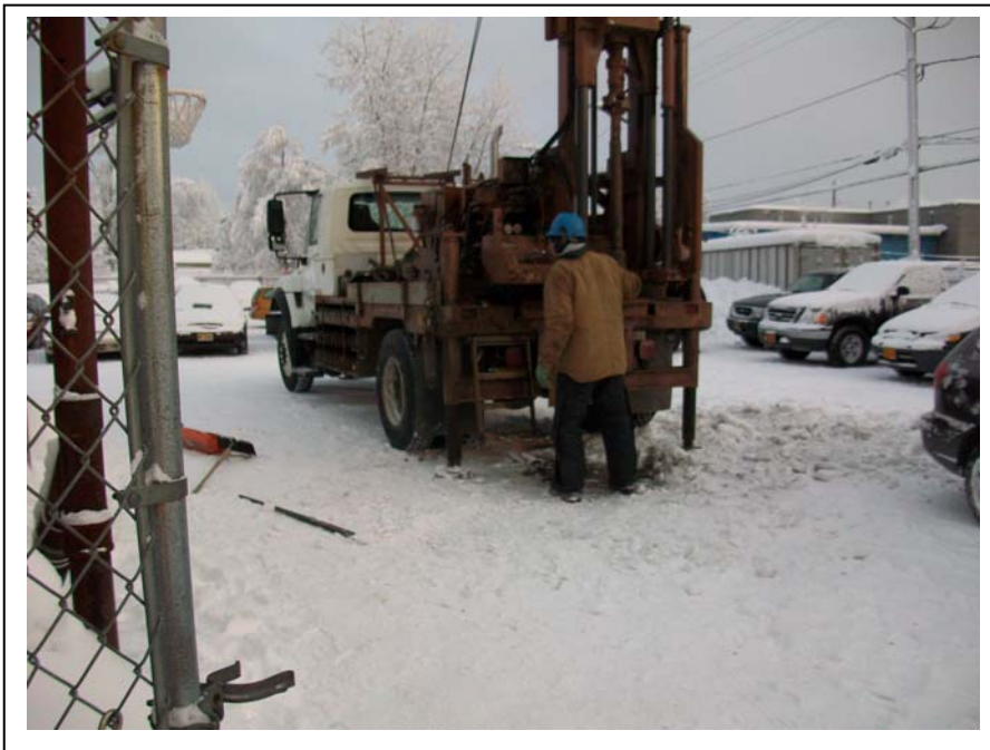
Photograph 2: Looking east, Vapor Extraction Well VE-2 was decommissioned by overdrilling, and filling the borehole with bentonite chips. (December 18, 2009)
