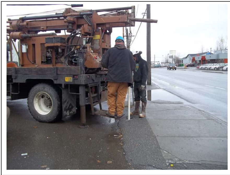
Photograph 1: Looking north, removing the well casing from Monitoring Well MW-5 (October 17, 2011).
