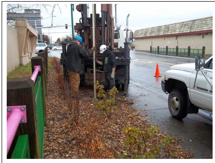
Photograph 2: Looking east, removing the well casing from Monitoring Well MW-7. (October 17, 2011).
