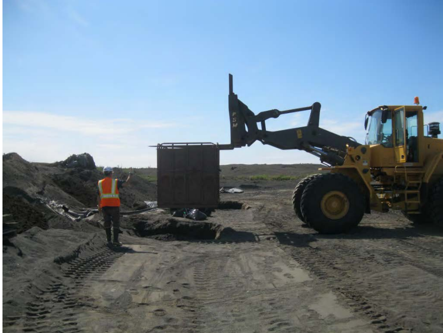
Photo No. 1 – 27 July 2013
