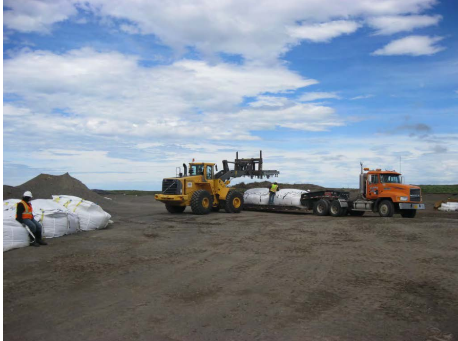
Photo No. 6 – 31 July 2013
