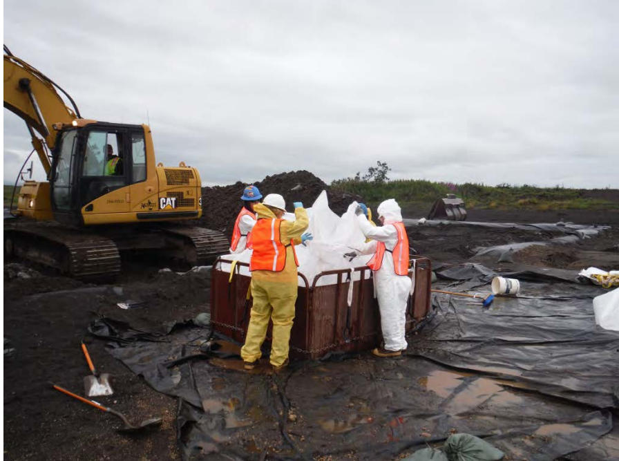
Photo No. 10 – 16 August 2013
