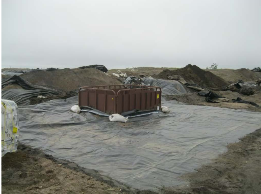
Photo No. 2 – 27 July 2013
