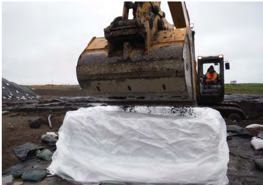
Photo No. 4 – 17 August 2013 Excavator filling bag from Stockpile J 1.4, looking west.
