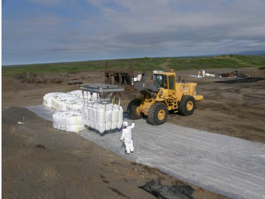
Photo No. 5 – 27 July 2013
