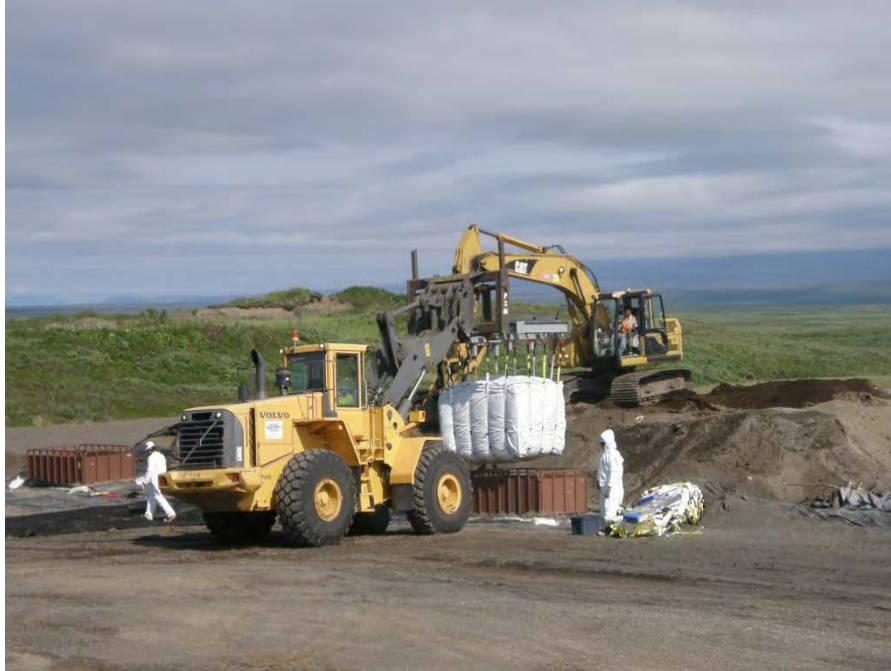
Photo No. 3 – 27 July 2013 Loader lifting a bag full of soil out of frame at Storage Area CA 1, looking northeast.
