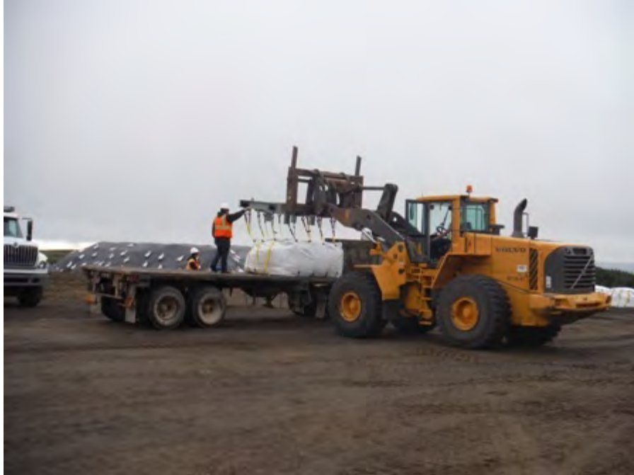
Photo No. 9 – 15 August 2013
