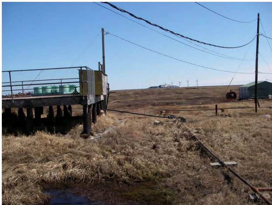
PHOTO 5: VIEW TO NORTHEAST FROM SOUTHWEST CORNER OF SITE
