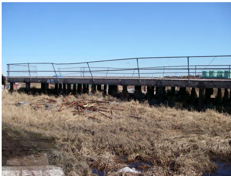
PHOTO 4: DEBRIS AND OLD TANK FARM DECK, VIEW TO THE NORTH FROM EAST SIDE OF SITE
