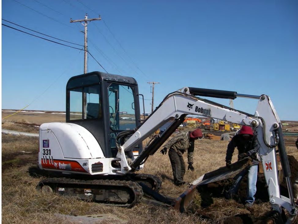
PHOTO 1: BACKHOE, OPERATOR, AND LABORER REMOVING DEBRIS BEFORE DIGGING TEST PIT TP-1, VIEW TO THE NORTH
