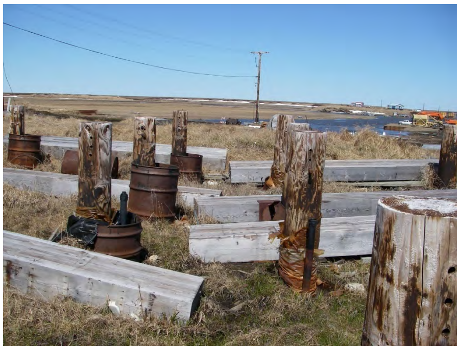
PHOTO 6: PILINGS FROM SMALLER OLD TANK FARM DECK AT NORTH CORNER OF SITE, VIEW TO THE NORTHEAST, TEST PIT TP-3 LOCATED TO THE RIGHT OF THE PHOTO
