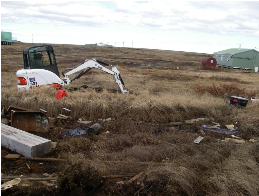
PHOTO 8: DIGGING TP-6 OUTSIDE OF BERM AT SOUTHEASTERN CORNER OF SITE; VIEW TO THE SOUTHEAST.
