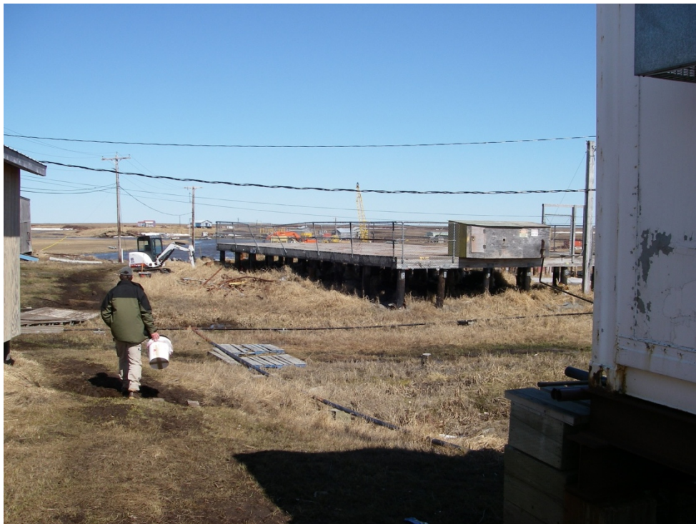
PHOTO 2: VIEW TO THE NORTH OF FORMER TANK FARM DECK
