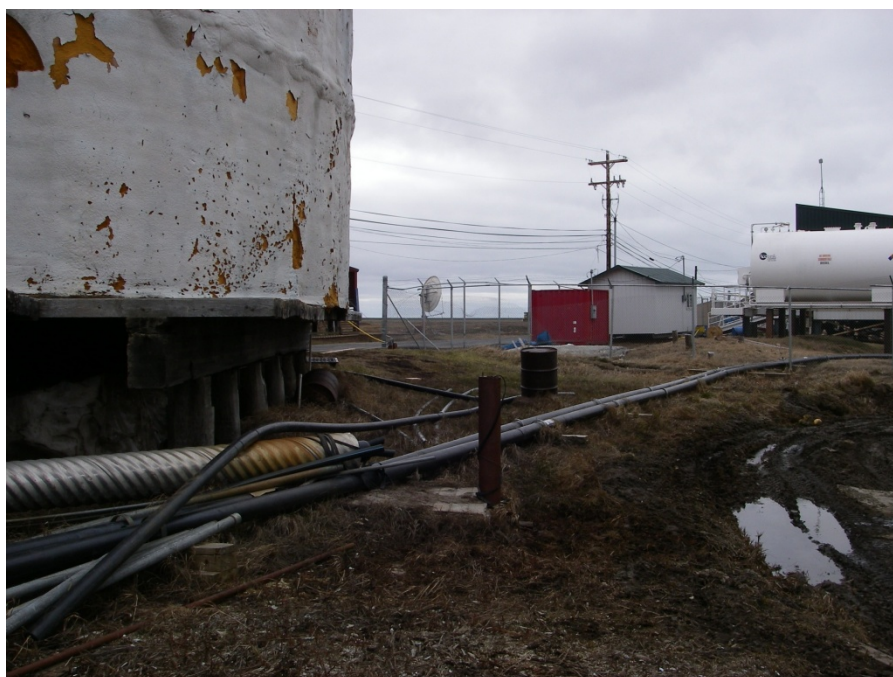
PHOTO 10: CASING IN CENTER OF PHOTO IS OLD WELL LOCATED NEAR WASHETERIA, APPROXIMATELY 350 FEET SOUTH OF THE FORMER SCHOOL TANK FARM, VIEW TO THE NORTH
