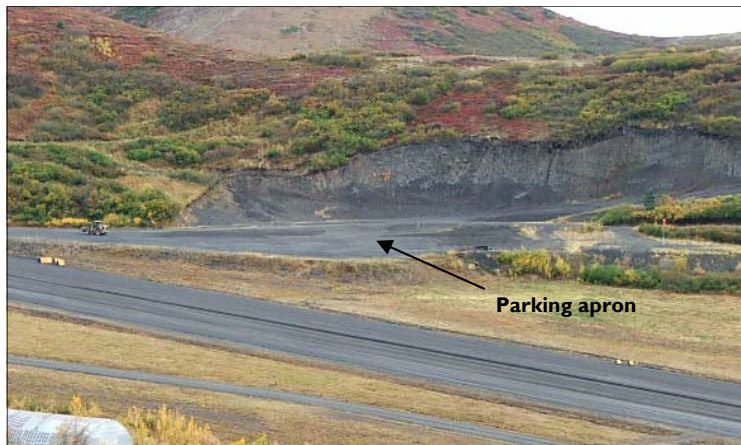
Looking northeast at SS007 with the runway in the foreground (2006).
