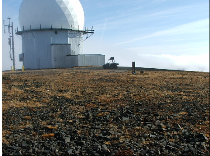
Looking east across area affected by diesel spill at ST006 (2006).
