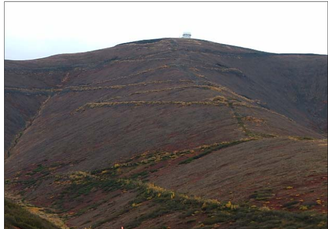
Abandoned switchback road to Upper Camp looking north with the radome in the background (2006).
