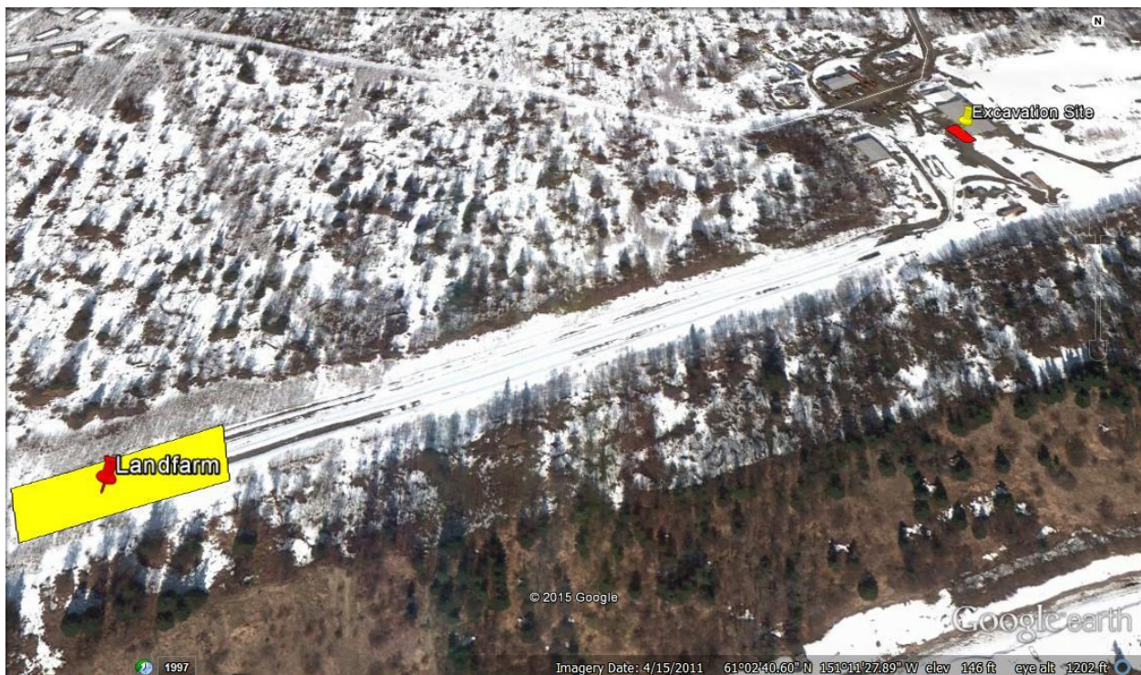
Figure 4 – The constructed landfarm site relative to the excavation site.
