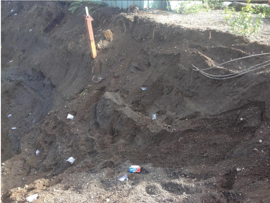
Photo 5 – Field screen and laboratory sample locations. Boring B-1 from 1998 ESA and the electrical power cables are visible in the photograph.
