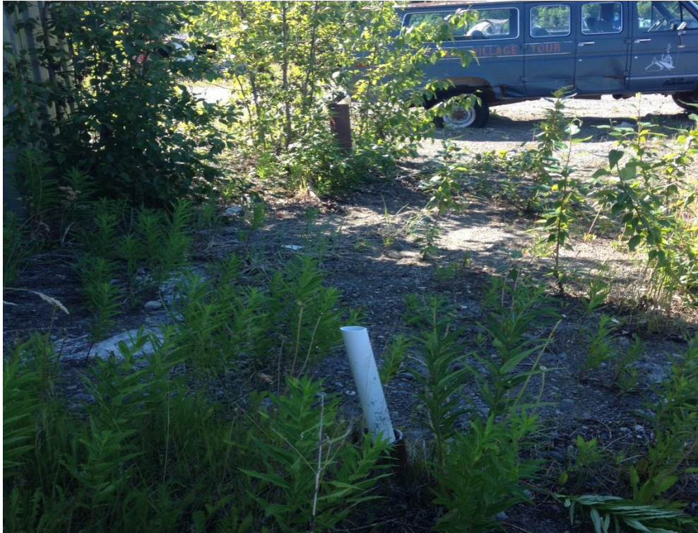
Photo 2 – Old air sparging placed in the original borings from the 1998 ESA.
