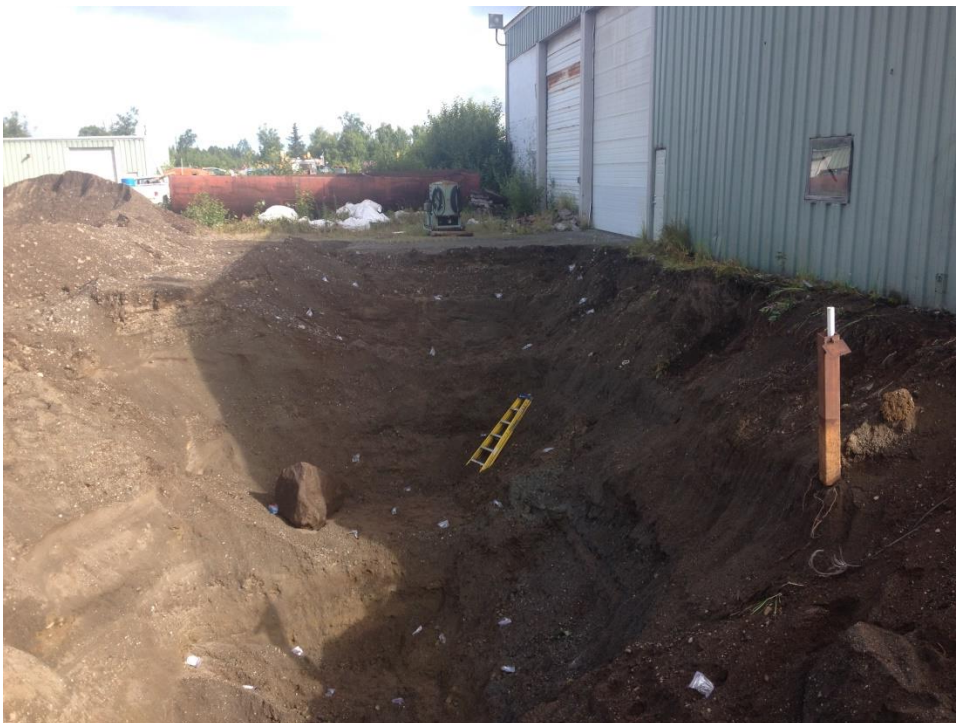
Photo 4 – Confirmation field screen sampling in the tiered excavation.
