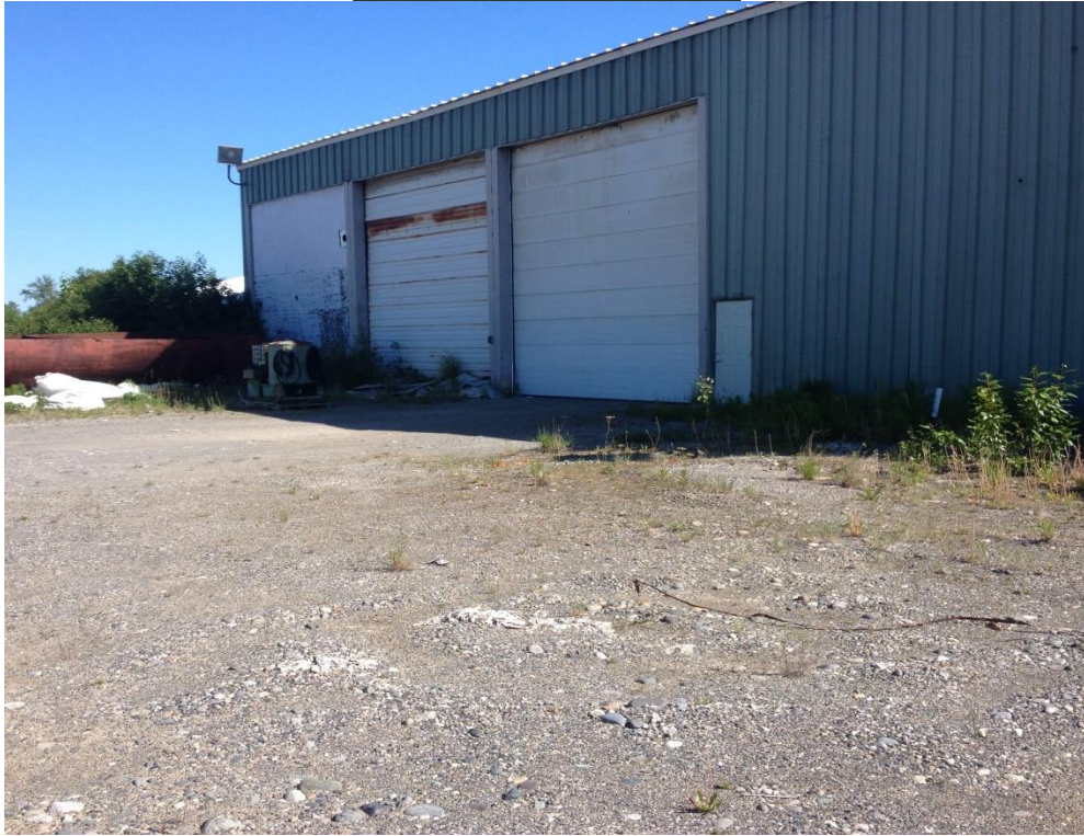
Photo 1 – site prior to excavation work
