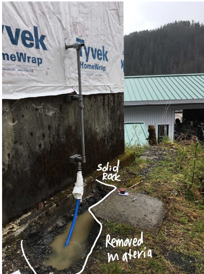
Figure 9. Workshop and generator shed area: Removed material.
