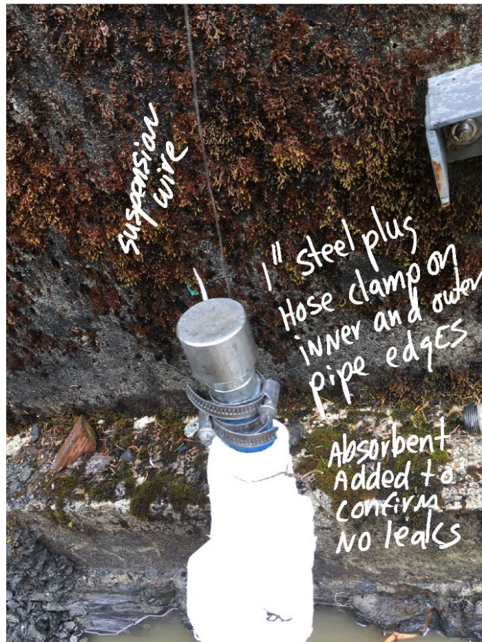
Figure 10. Workshop and generator shed area: Ahtna repairs.
