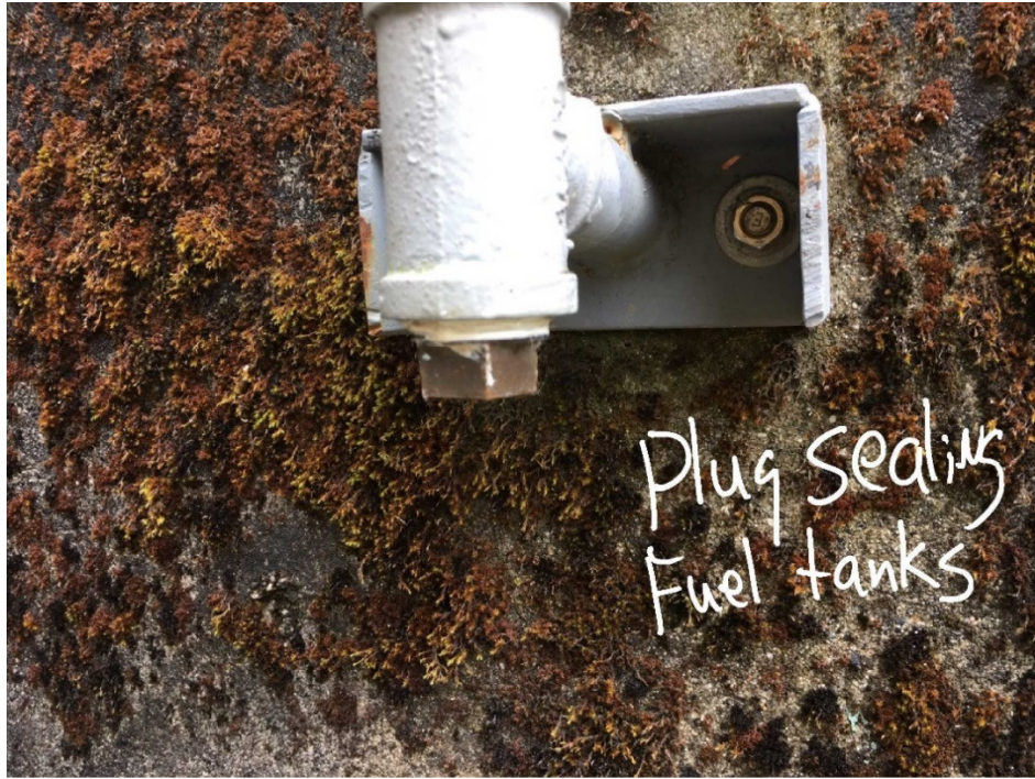
Figure 9. Workshop and generator shed area: Ahtna repairs.
