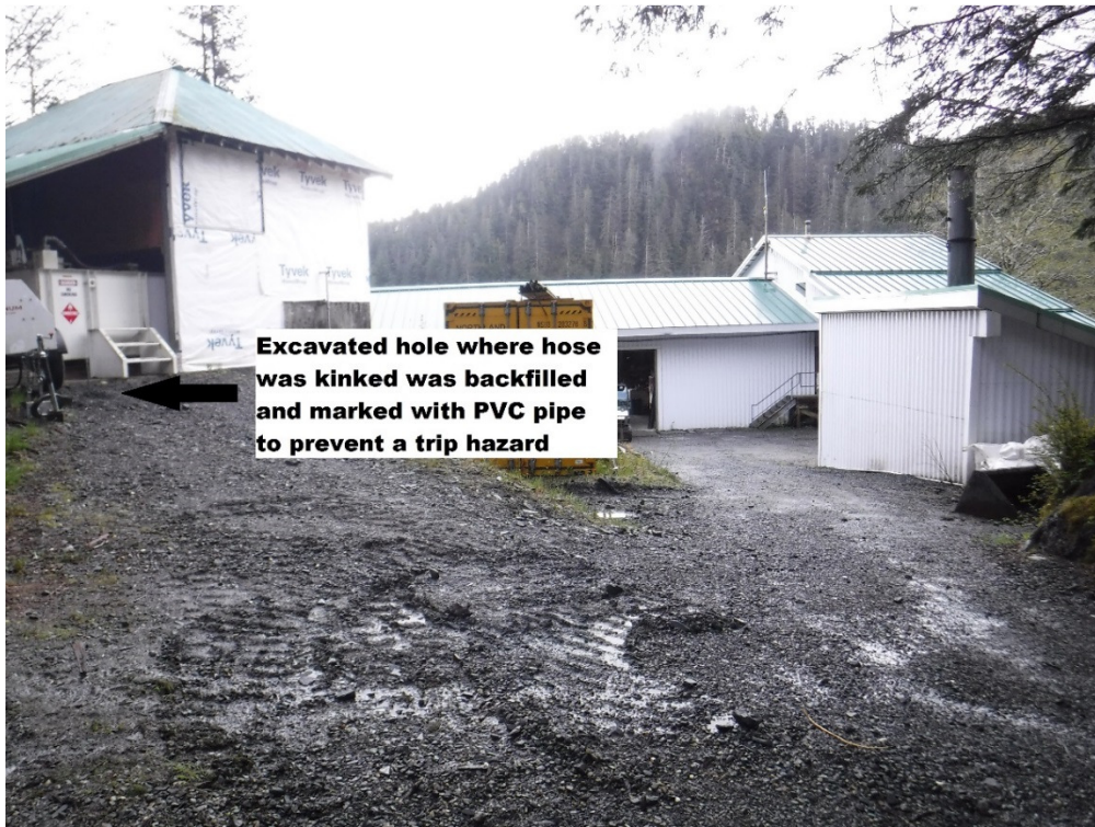
Figure 13. Workshop and generator shed area: Backfilled areas.
