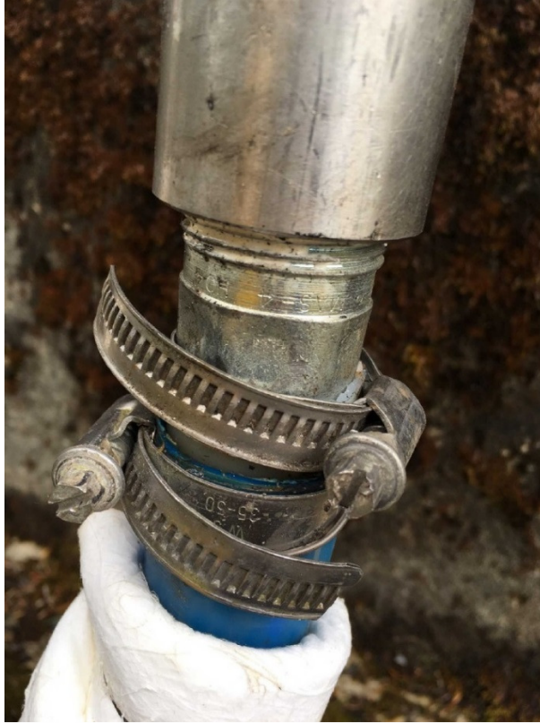
Figure 11. Workshop and generator shed area: Ahtna repairs.
