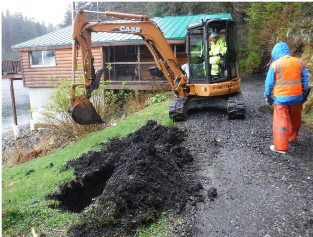
Figure 13. TPH soil investigation at the Pan Abode Cabin
