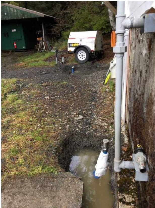
Figure 12. Workshop and generator shed area: Ahtna repairs to both locations.
