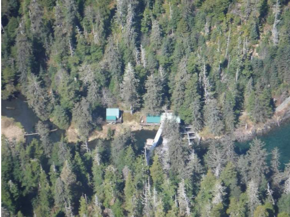
Figure 2. Aerial photo of Weir Cabin and Pan Abode Shop
