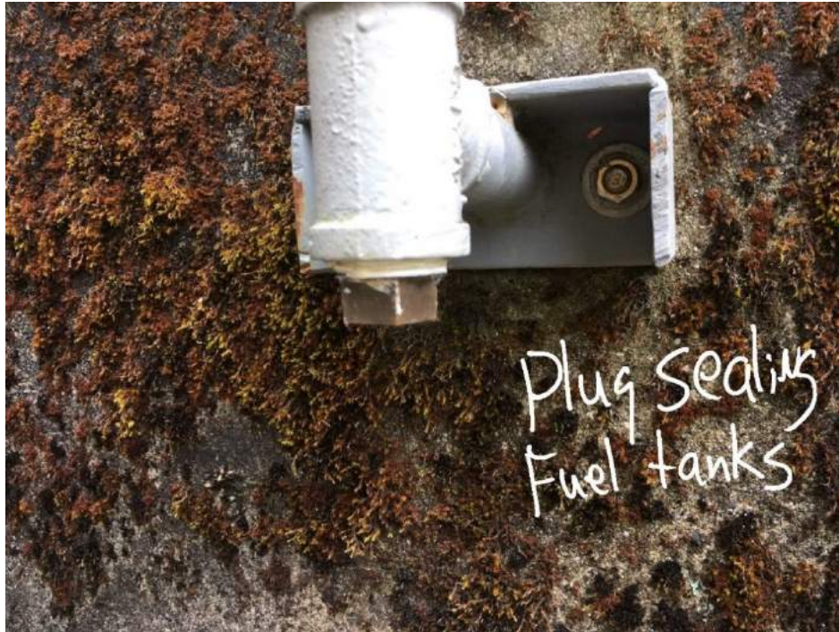
Figure 9. Workshop and generator shed area: Ahtna repairs.
