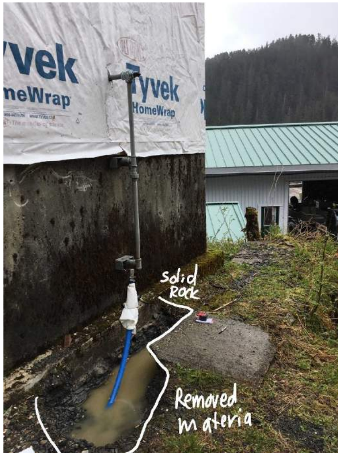
Figure 9. Workshop and generator shed area: Removed material.
