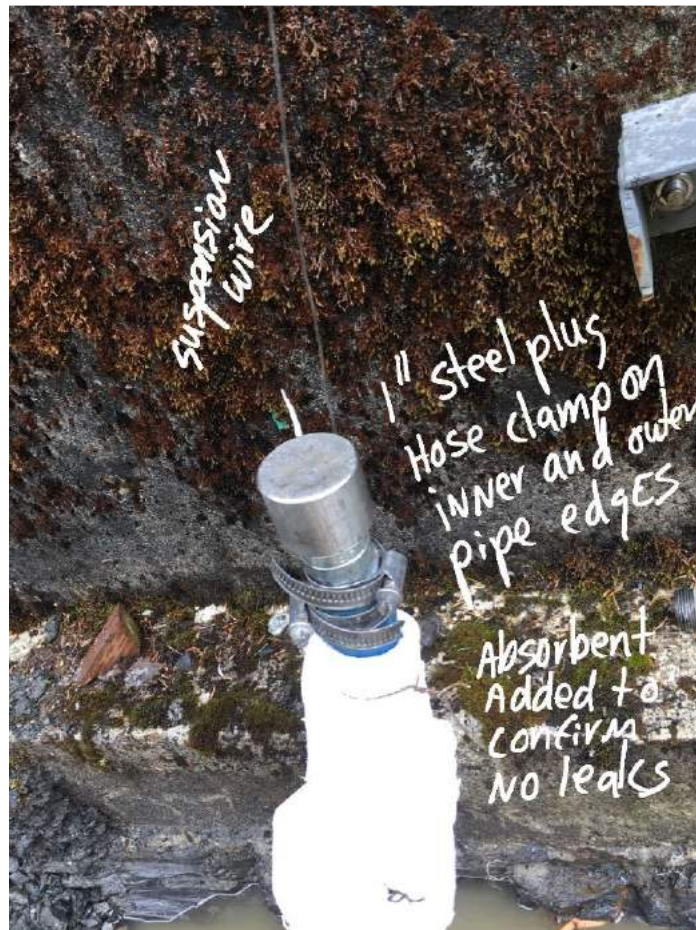
Figure 10. Workshop and generator shed area: Ahtna repairs.
