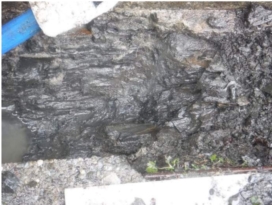
Figure 10. Workshop and generator shed area: Removed material to bedrock.
