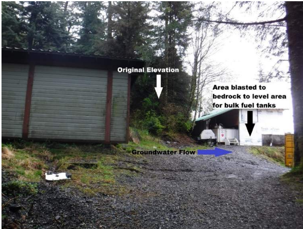
Figure 1. Workshop and generator shed area: Blasted bedrock to build structures.
