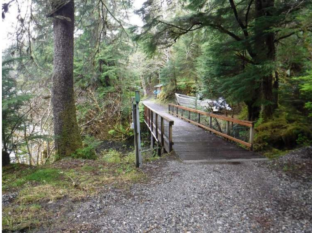
Figure 8. Bridge constructed of pressure treated lumber
