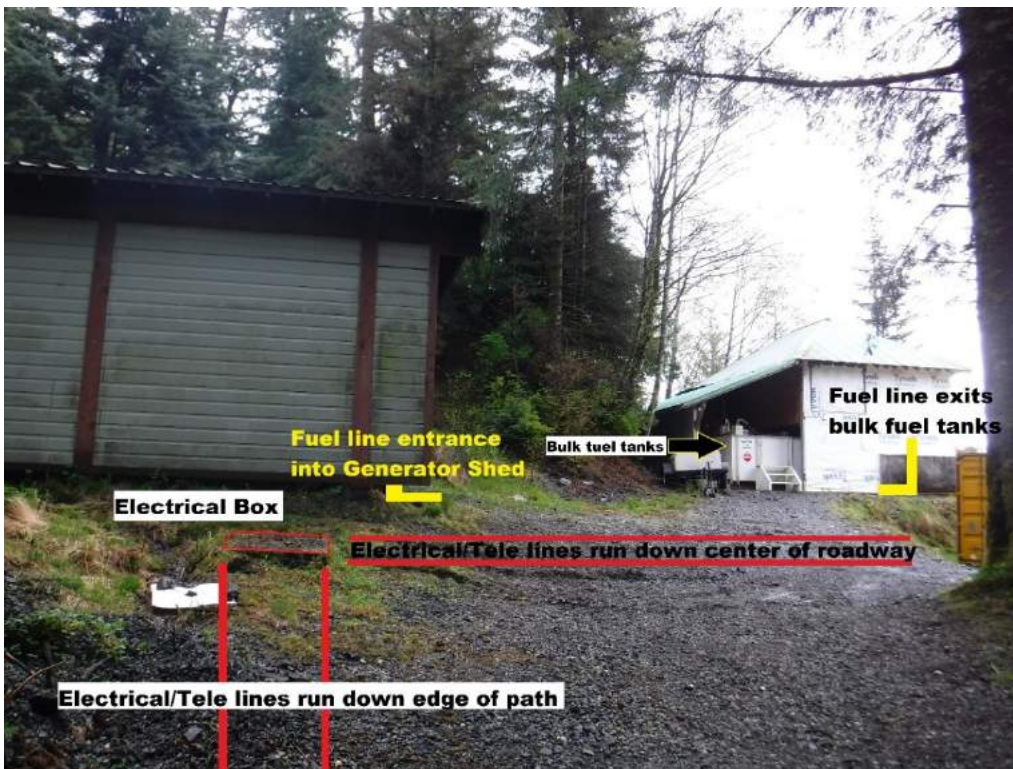
Figure 2. Workshop and generator shed area: Utility locations.
