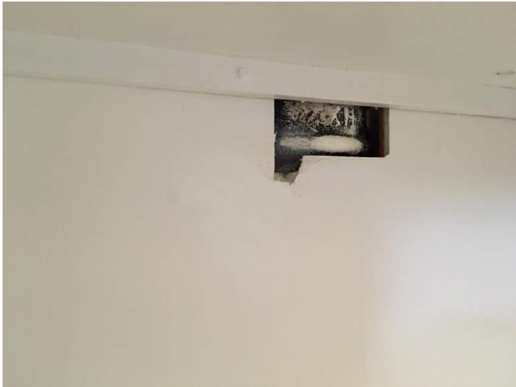
Figure 11. ACM sample location of bathroom drywall in White House
