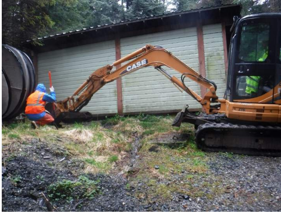
Figure 3. Workshop and generator shed area: Ahtna operator and spotter.
