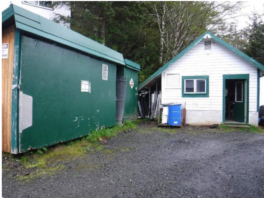
Figure 7. HazMat Shed and Work/Metal Shop
