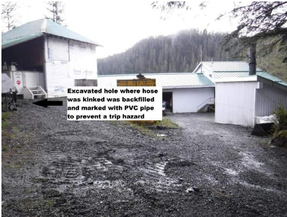
Figure 13. Workshop and generator shed area: Backfilled areas.
