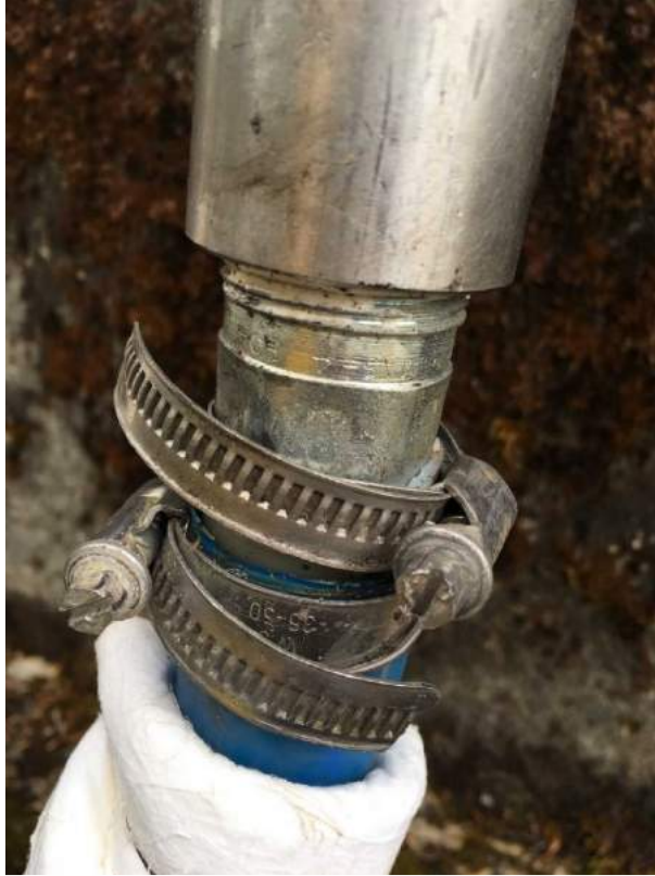
Figure 11. Workshop and generator shed area: Ahtna repairs.
