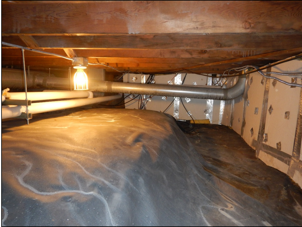
Photograph 13: Crawlspace vapor barrier. Looking east.
