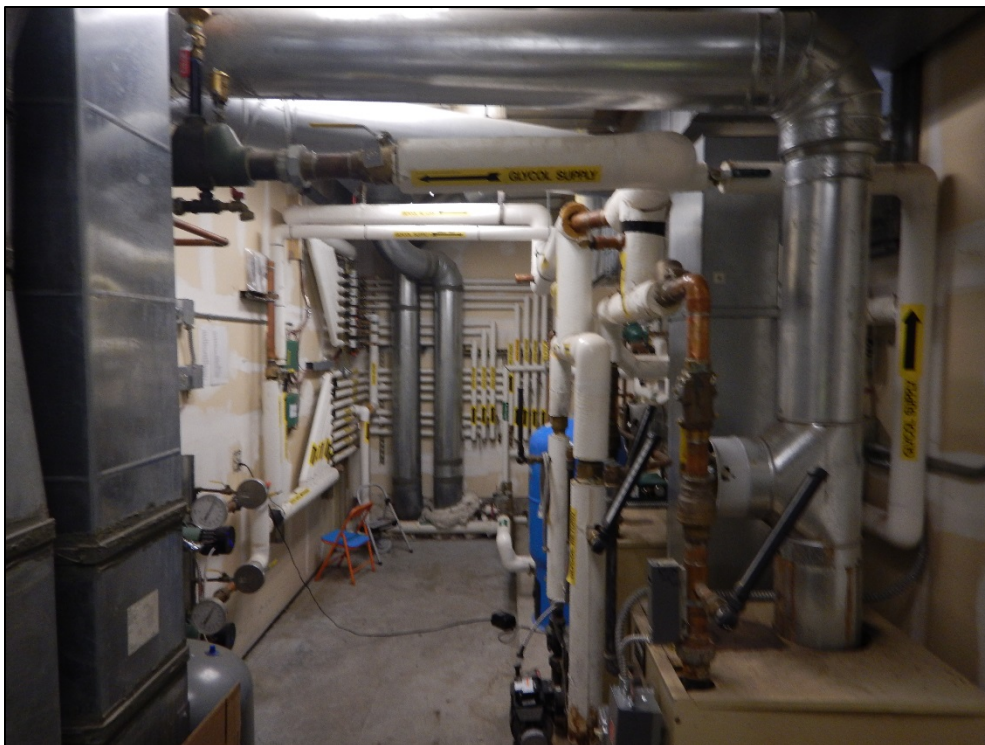
Photograph 6: Furnace room. Looking east.
