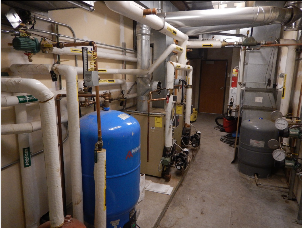
Photograph 7: Furnace room. Looking west.
