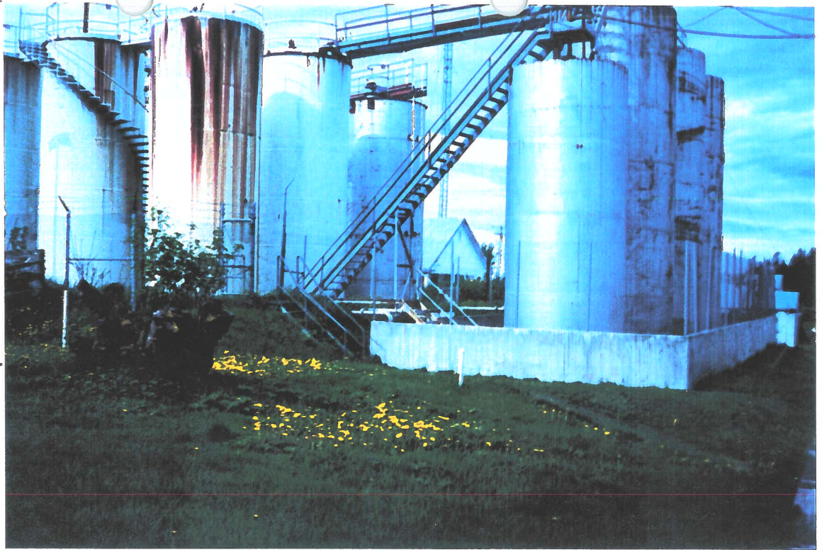
ORIGINAL TANK FARM WITH EARTHEN BERM & EXPANSION WITH CONCRETE CONTAINMENT
