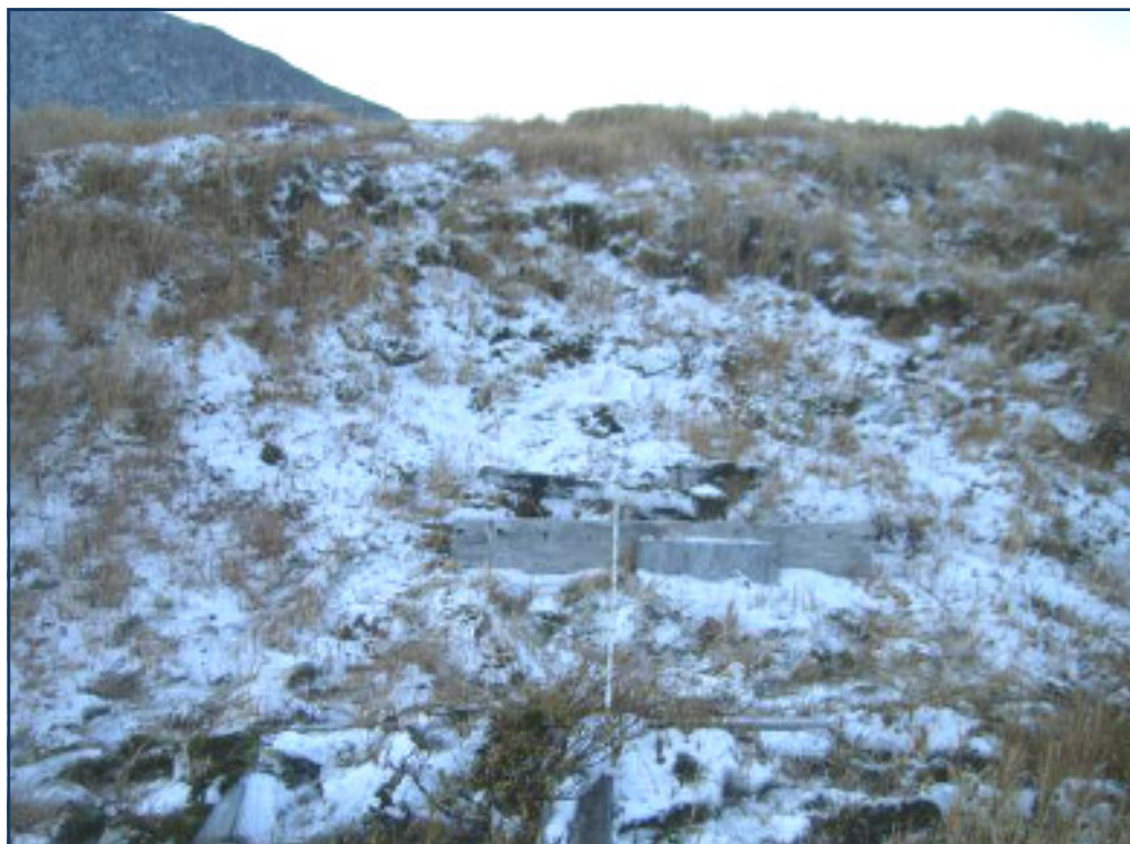
Concrete Target Foundations
