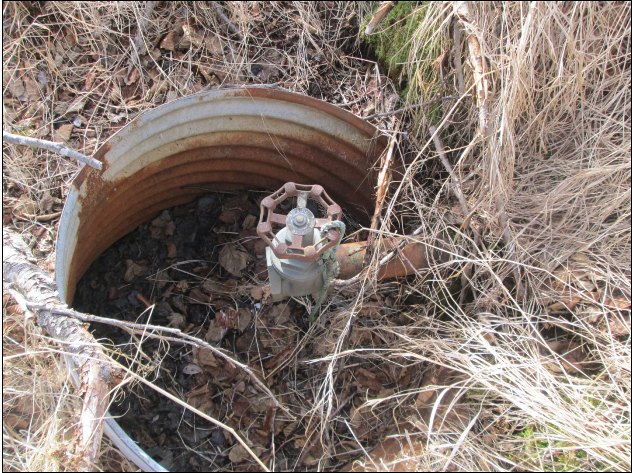
Figure 7. Pipe and valve assembly prior to removal.
