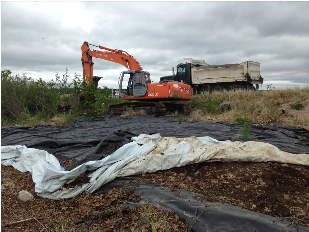
Figure 3. Removal of top liner from the bio-cell.
