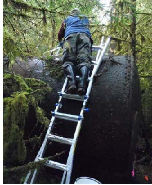
Photo 4: Inspecting AST within Fuel Storage Area, facing north (USACE, 2013)
