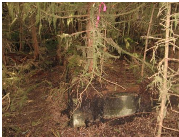
Photo 1: Power Plant concrete foundation, facing south (USACE, 2014)
