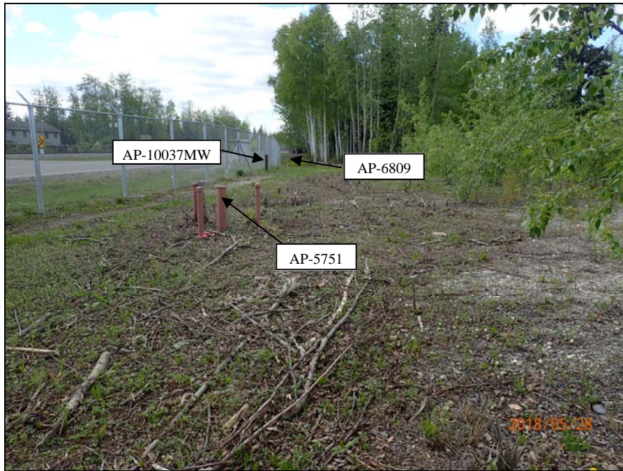
Building 1168 Leach Well monitoring wells (view to the W)
