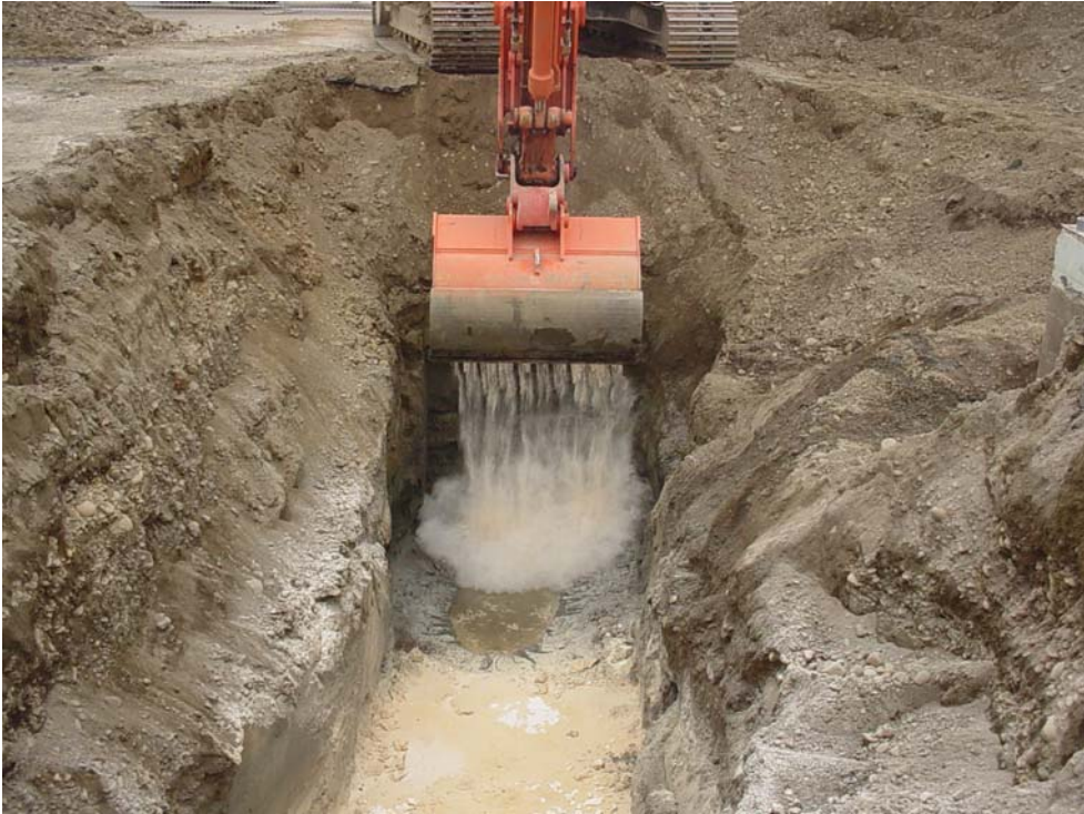
Photograph A2-3: Placing ORC-A in excavation.
