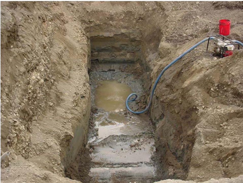
Photograph A2-2: Pumping hydrocarbon and groundwater emulsion.
