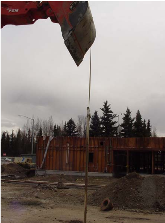
Photograph A2-2: Removal of casing and screen from MW-3a.
