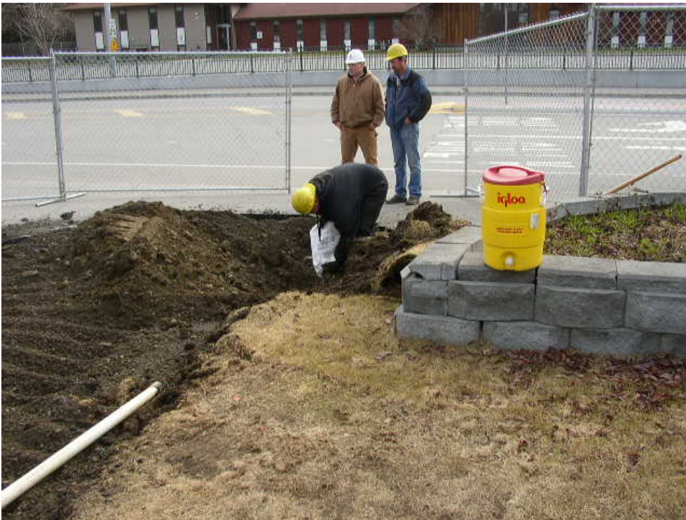
Photograph A2-8: Placing bentonite chips in hole, MW-4.
