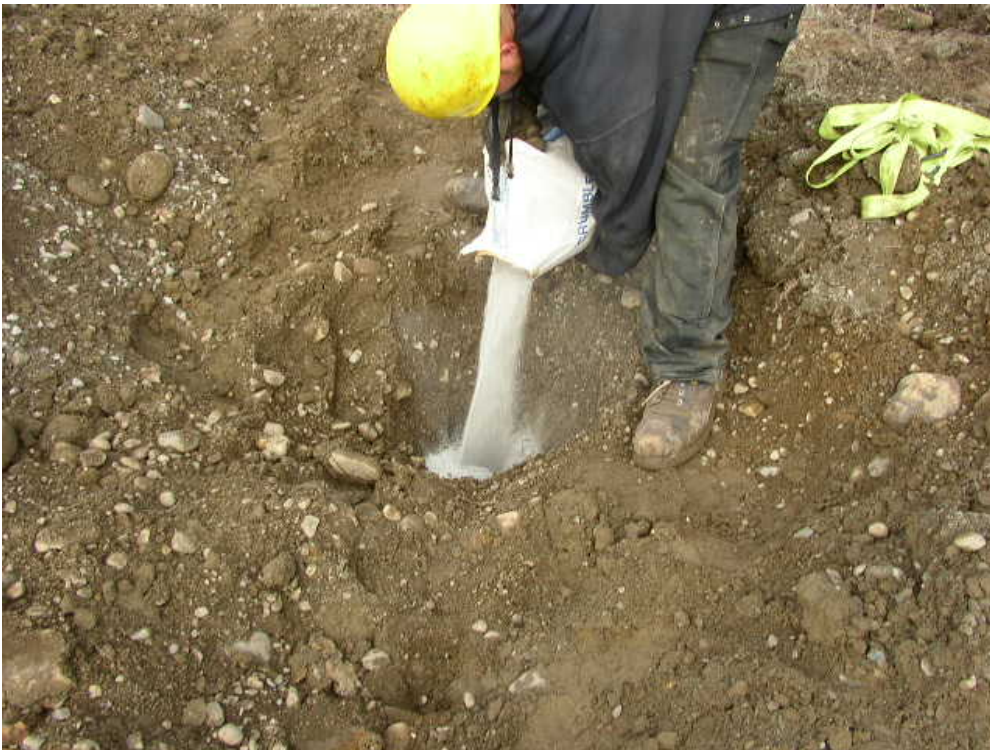
Photograph A2-6: Placing bentonite chips in hole, MW-2.
