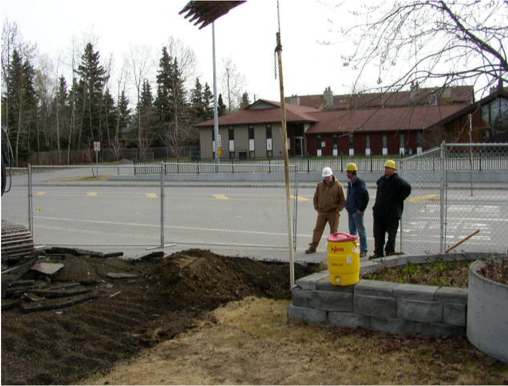
Photograph A2-7: Removal of casing and screen from MW-4.
