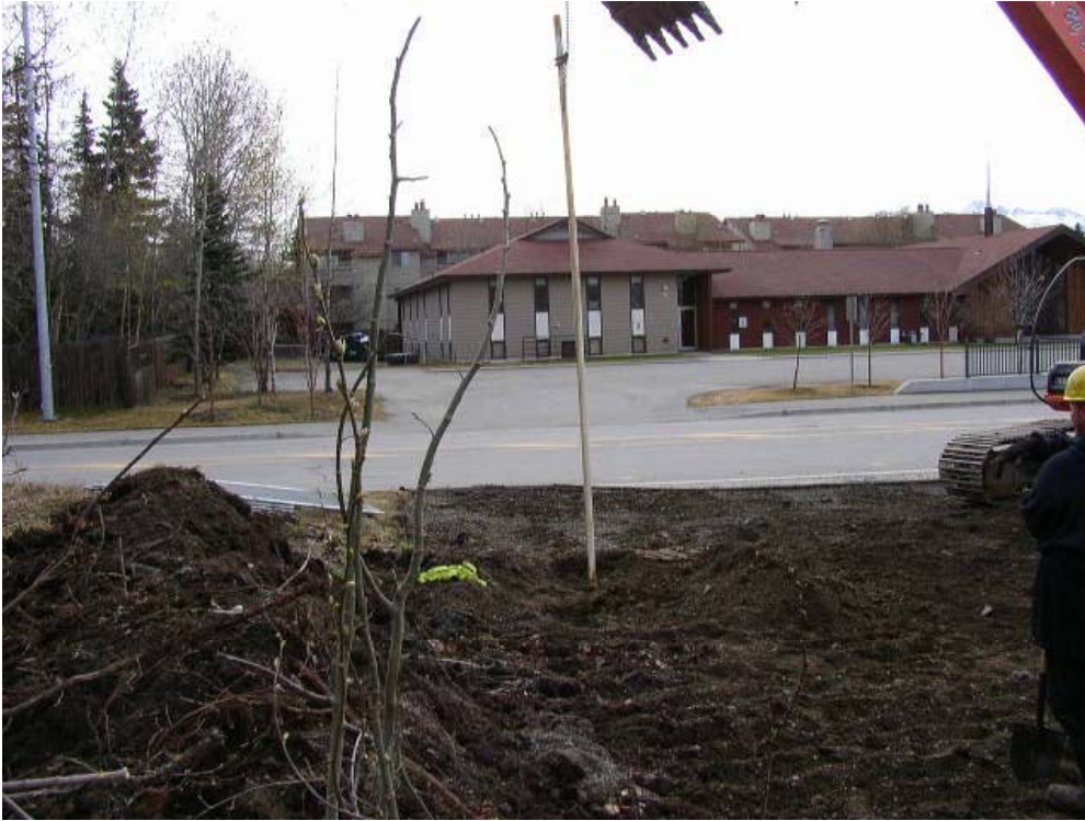
Photograph A2-5: Removal of casing and screen from MW-2.
