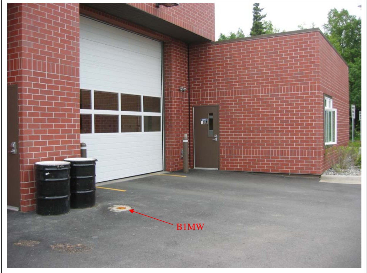
Photo 1: A view of Monitoring Well B1MW, located on the east side of Fire Station No. 4 after completion of installation; looking northwest (July 2008).
