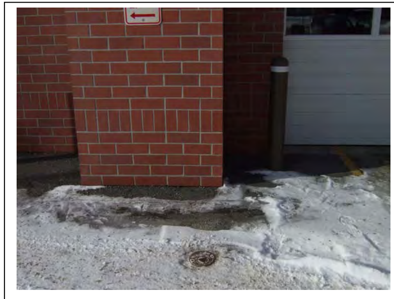
Photo 8: Looking west, a view of existing Well B1MW, located on the eastern side of Fire Station No. 4. (February 27, 2013)
