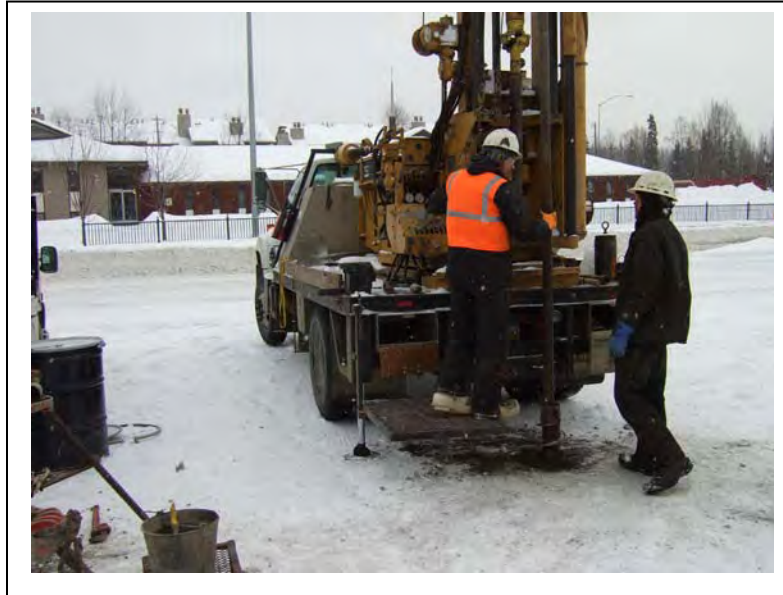
Photo 1: Looking east, a view of Discovery Drilling drilling Boring B2. (February 22, 2013)
