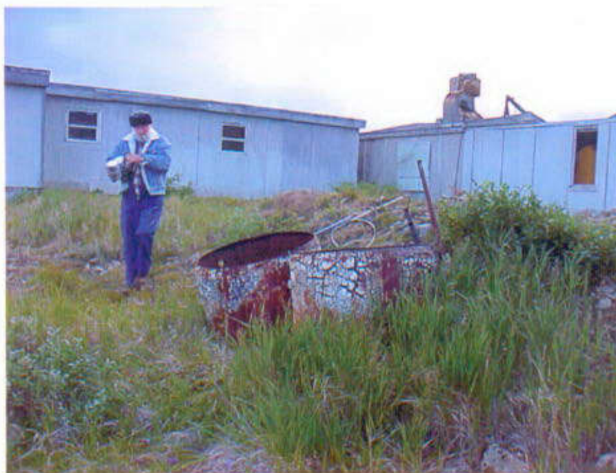
Photograph 3. A view of the septic man-ways above the septic tank behind building #4100 (the old weather station).
