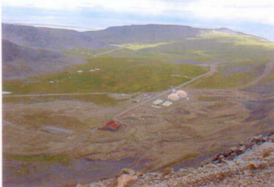
Photograph 1. A view of lower camp looking west. A biocell soil treatment cell, cold storage building, fuel storage and domes are visible in the foreground. One mile beyond the domes, on the left hand side of the road, is LF-003. The end of the runway is visible at the end of the road.
