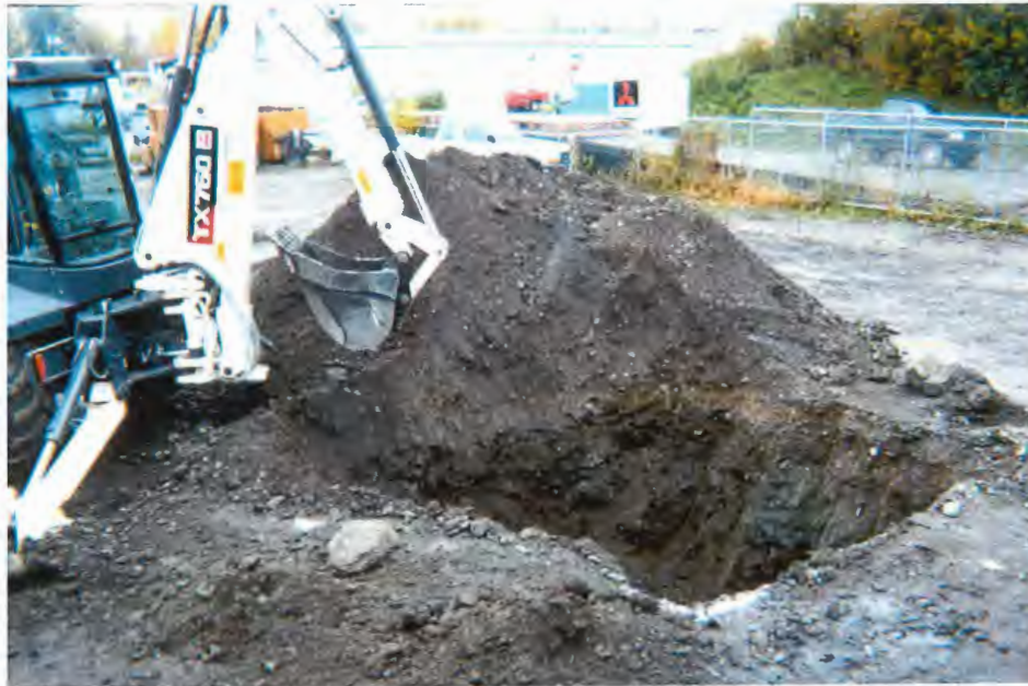
Photo 1: Looking southwest at Excavation 1.
