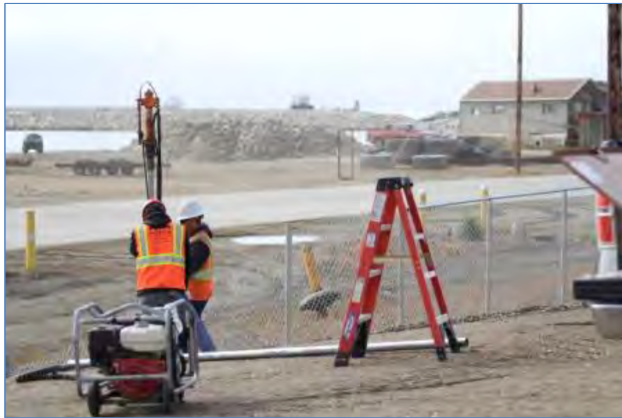
Photo No. 22 – 19 July 2016 Reinstallation of fencing. Looking southeast.
