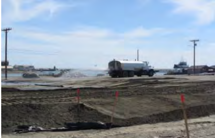
Photo No. 19 – 14 July 2016 Watering cap for compaction. Looking east.
