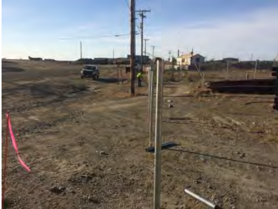
Photo No. 1 – 2 October 2015 Installation of fencing at the site. Looking southwest.
