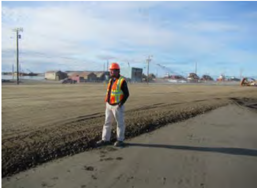
Photo No. 20 – 14 July 2016 Addition of two-inch minus gravel layer. Looking southeast.
