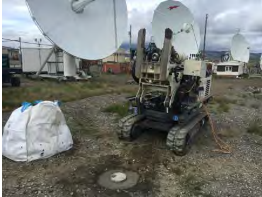
Photo No. 9 – 18 June 2016 W-36 completed as flush-mount monitoring well. Looking north.
