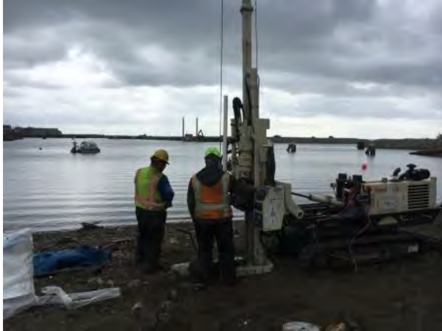
Photo No. 11 – 19 June 2016 Installing monitoring well W-37. Looking east.
