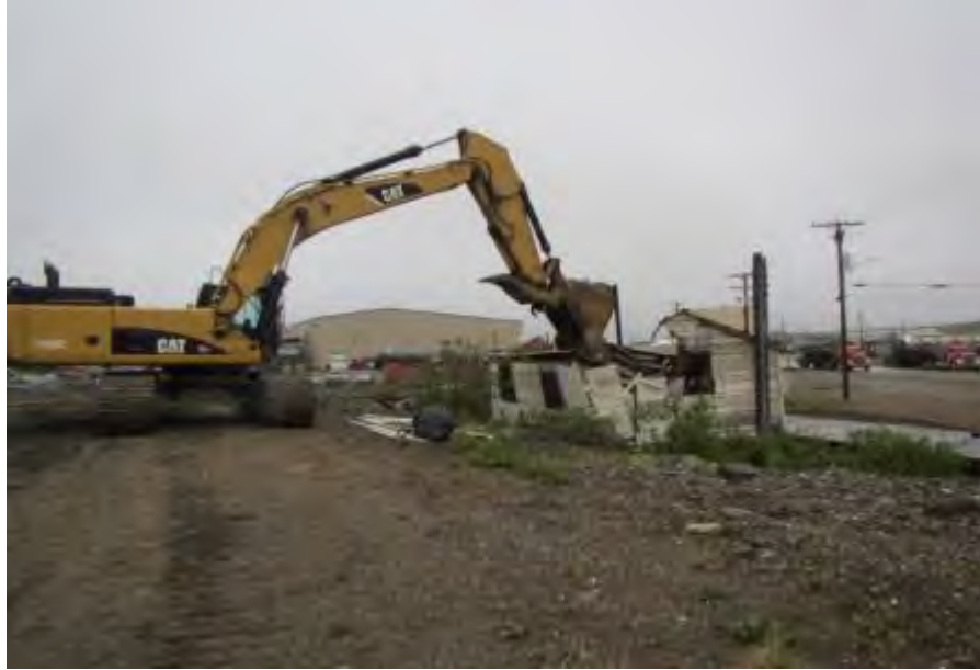
Photo No. 15 – 26 June 2016 Demolition of the old pumphouse. Looking northeast.
